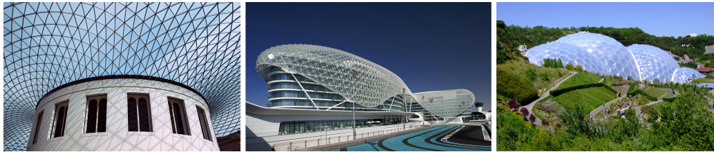
Figure 2.1 – The three types of gridshells. Triangular (left), British museum courtyard by Foster and Partners. Quadrilateral (center), Yas Hotel Abu Dhabi by Asymptote Architecture. Hexagonal (right), Eden project by Nicholas Grimshaw.
