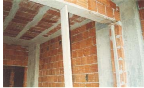
Figure 72_Example of the ceiling during a construction
