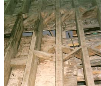
Figure 13_Bağdadi System Example
