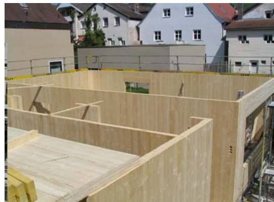
Figure 46_CLT element application example
