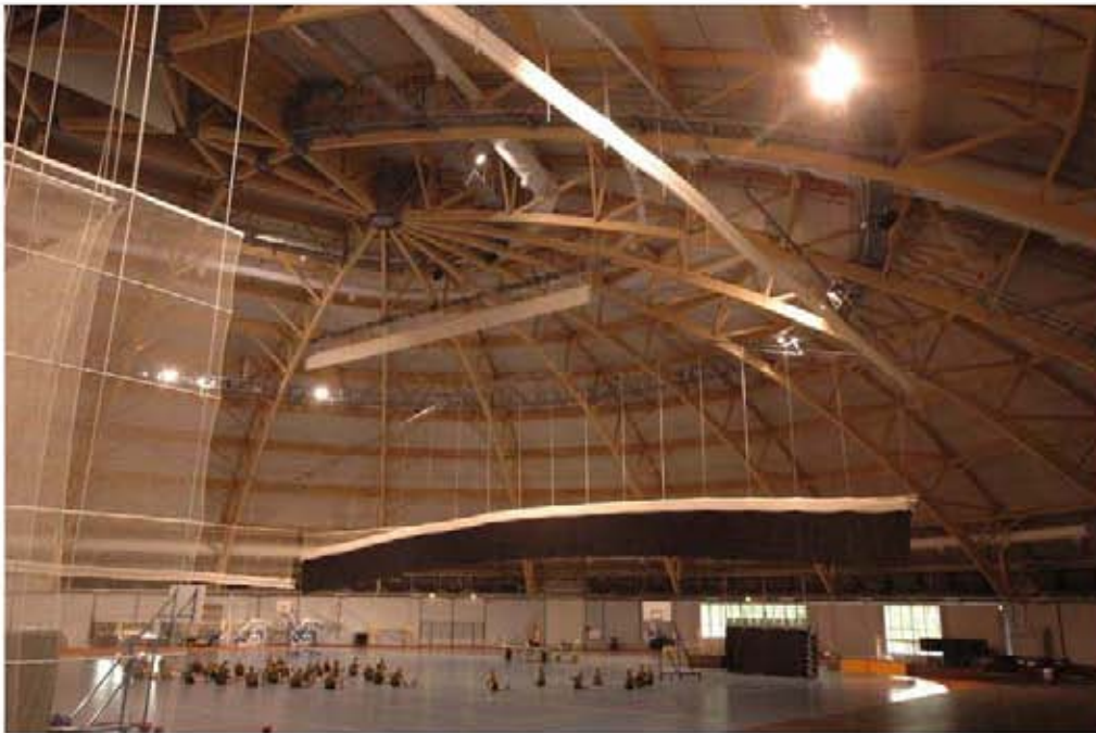
Figure1.1. An example of a large span wooden building Multi-purpose Arena, Joensuu, Finland, 2006
