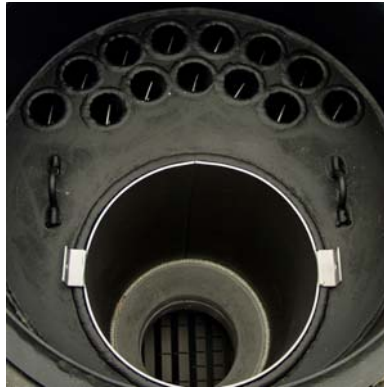
Figure 4: Exchangeable bush in the heat exchanger
