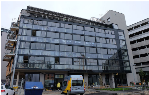
Figure 1. The Bikes and Rails building. Source: authors' own.
