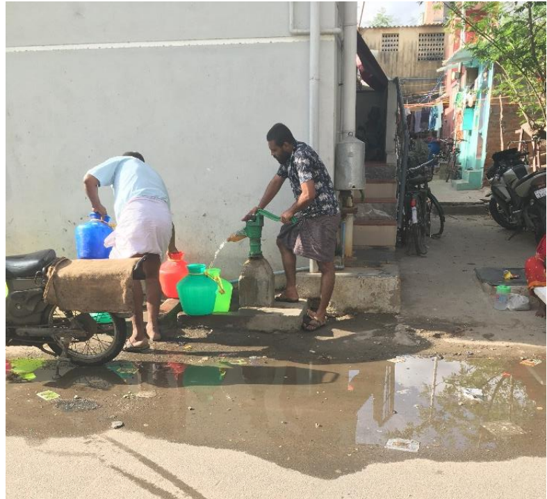
Picture 53: Metro water tap on the street. Source: own Photograph
