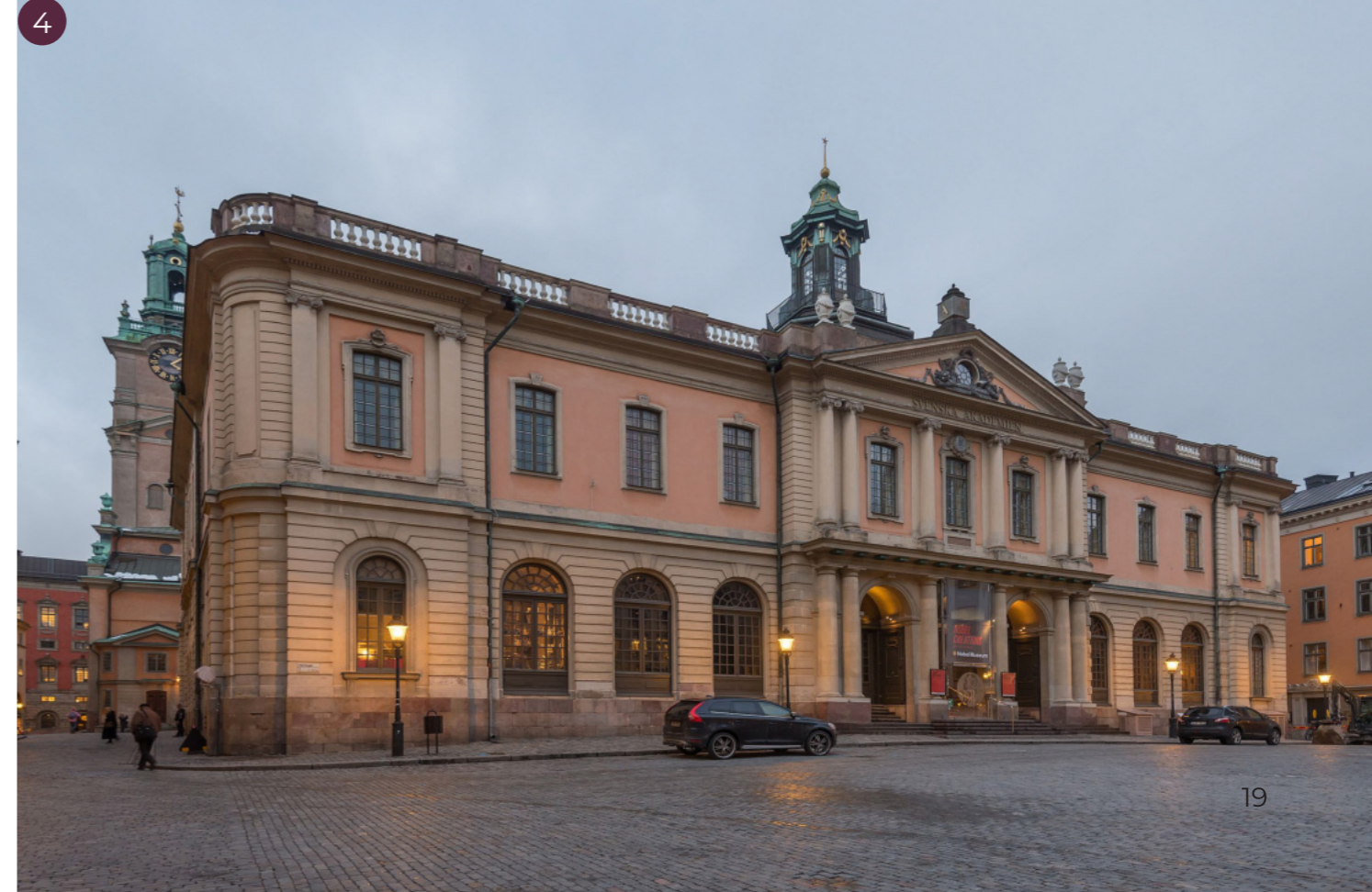
4 Ill. 9. The Stock Exchange Building
