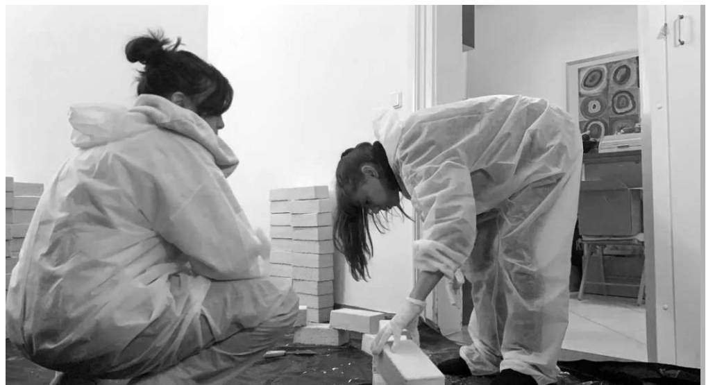
Figure 36 building the pavilion
