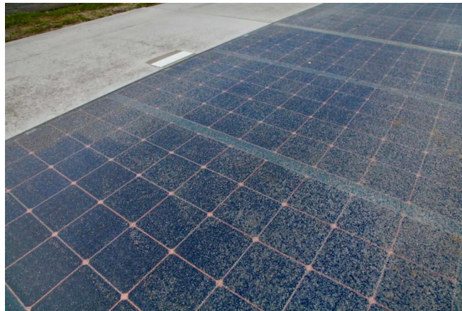
Figure 3.2 - SolaRoad photovoltaic surface [3333]
