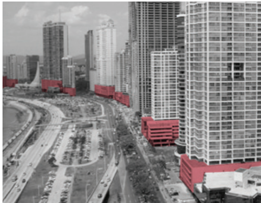
Abb. 28 - Parketagen in der Sockelzone, Cinta Costera [2016]
