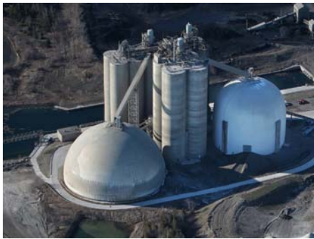
FIGURE 18: Rotatorially symmetric concrete dome built by Dome Technology [21] ©Dome Technology.
