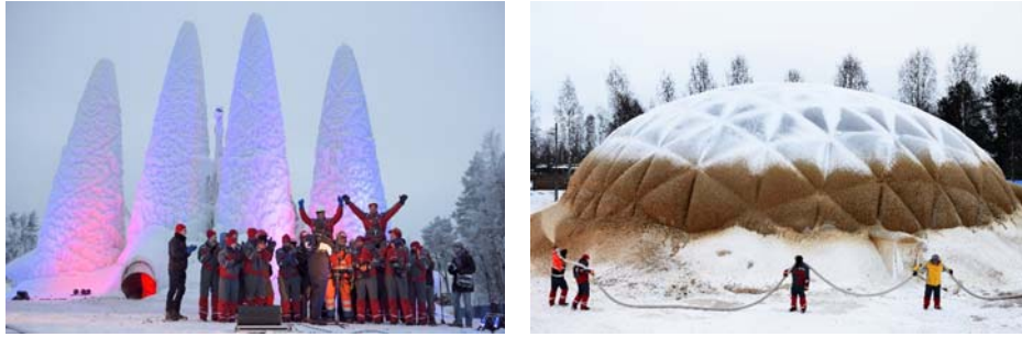
FIGURE 13: Ice structures built with pneumatic formwork by Pronk [17, 18].
