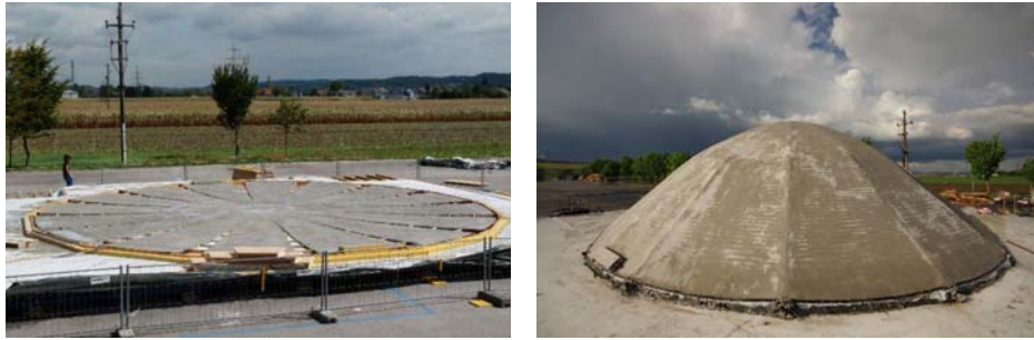
FIGURE 21: Large-scale experiment in Austria: erection of a spherical shell using PFHC (2012).
