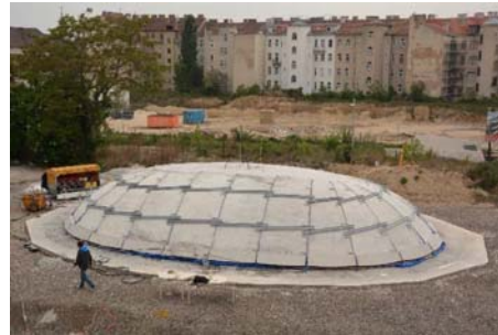
FIGURE 23: Large-scale experiment in Austria: erection of a free-form concrete shell using PFHC (2014).
