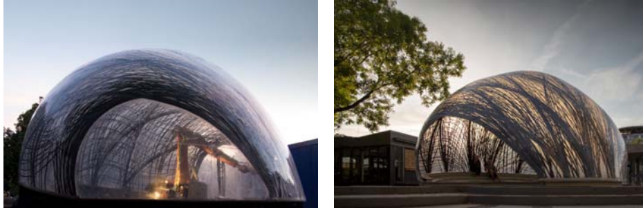
FIGURE 15: Inflated pavilion strengthened with carbon fibers which are applied by a robot arm [19] ©ICD/ITKE University of Stuttgart.
