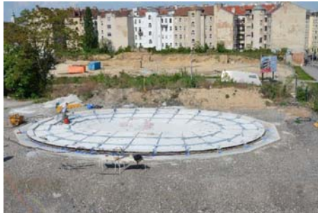
FIGURE 23: Large-scale experiment in Austria: erection of a free-form concrete shell using PFHC (2014).
