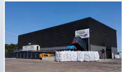
Exterior photo of the Green Carbon plant with the carbonized material filled in BIG BAGs filled carbonized material ©Polytechnik
