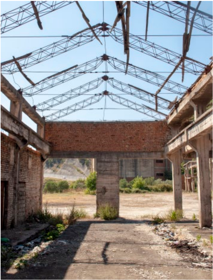
Steel trusses made of welded rebar create a filigree roof construction
