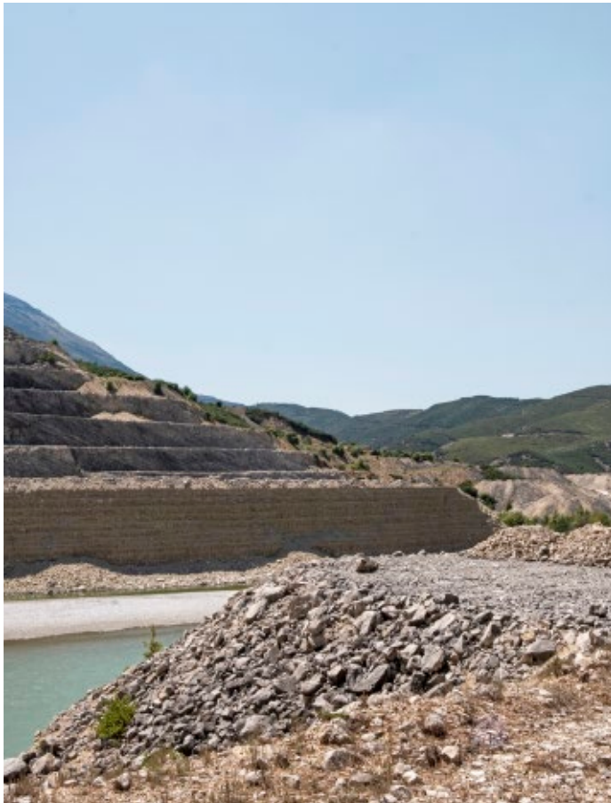
I Rocks and sand from the surrounding hills were used to create the 8 meter high platforms
