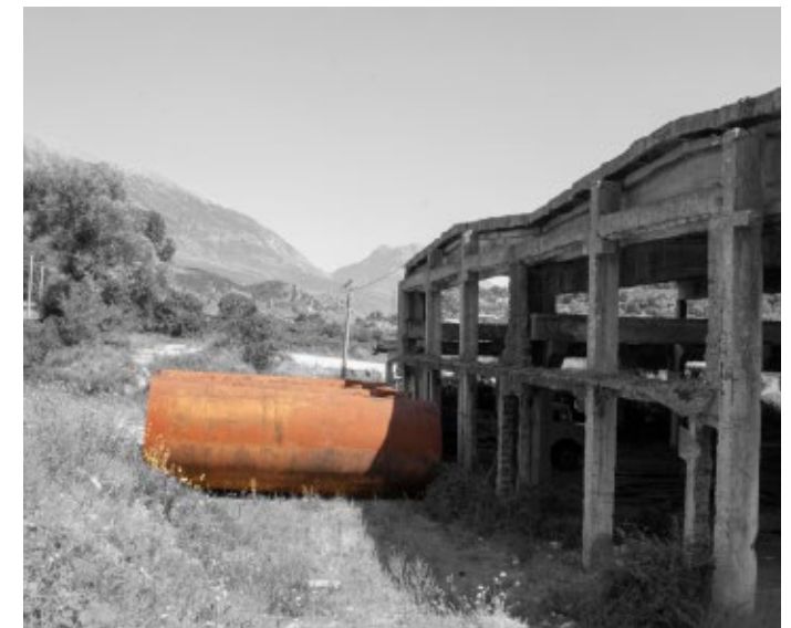
Old silos found on the site and pipes from the old factory are cut and used to create window openings
