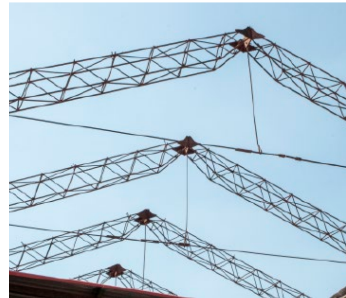
Steel trusses inspired by the beams at the old factory in Memaliaj are used for the construction of the roof, creating a double pitch
