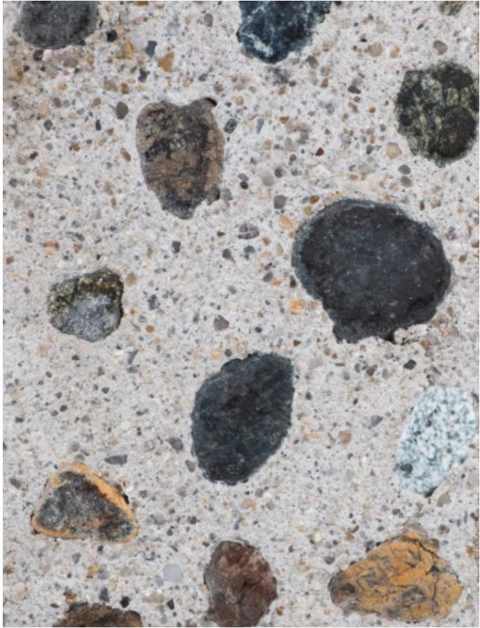
I The friction of the slabs is increased by washing out the surface to expose the riverstones and aggregate fo the Riverstone Concrete
