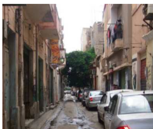
Figure.1.11: Exterior views of courtyard buildings
