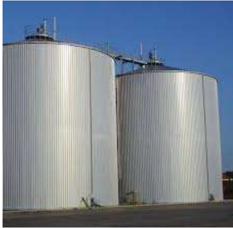
Figure 4 Two digesters at the waste water treatment plant of Bruck an der Leitha, Austria
