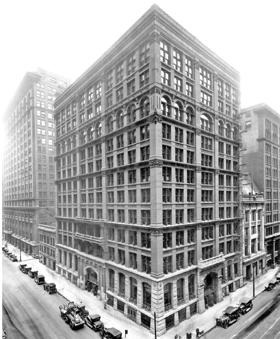
Abb. 167: Home Insurance Building in Chicago, Jenney, 1885
