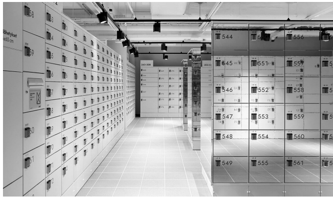
Pictures 71 shows BOX's locker system, the picture, the picture below automatic pick-up and drop-off stations.
