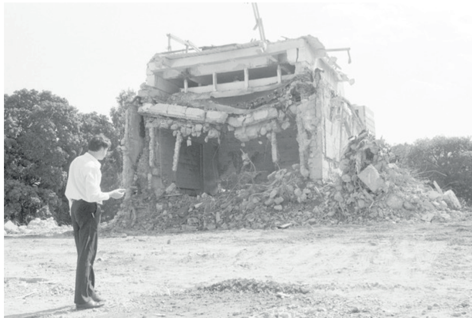
3 The demolition of Georgi Dimitrov Mausoleum in August 1999
