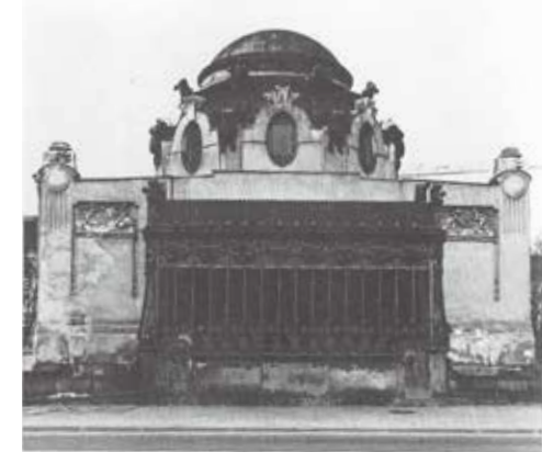
Abb. 5: Stadtbahn Station Schönbrunn, 1896
