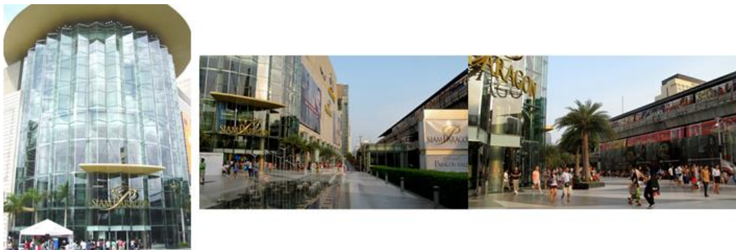
Figure 53 - Siam Paragon - Entrance and in-between spaces
