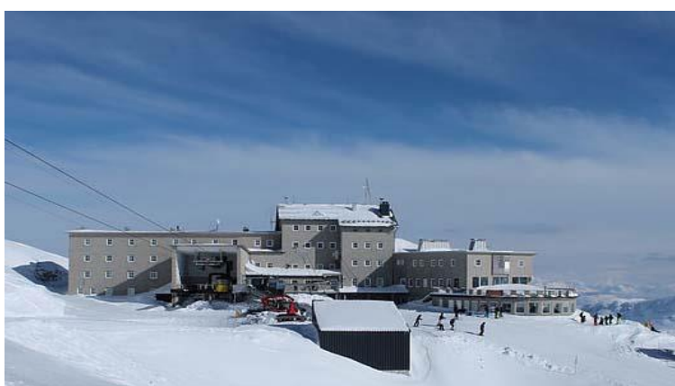
Figure 7. Krippenstein mountain base station before refurbishment (Source: Mein Bezirk 2015)
