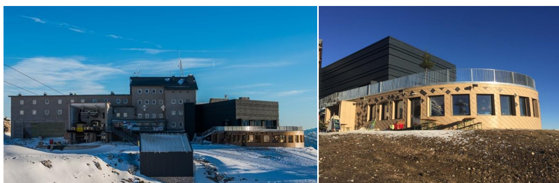
Figure 8. Krippenstein mountain base station after refurbishment (Source: Dachstein Salzkammergut 2016)
