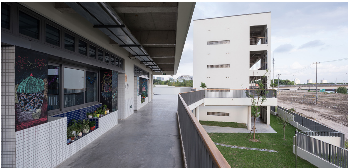
Ill. [45] Corridor at Tongji University Affiliate Elementary School
