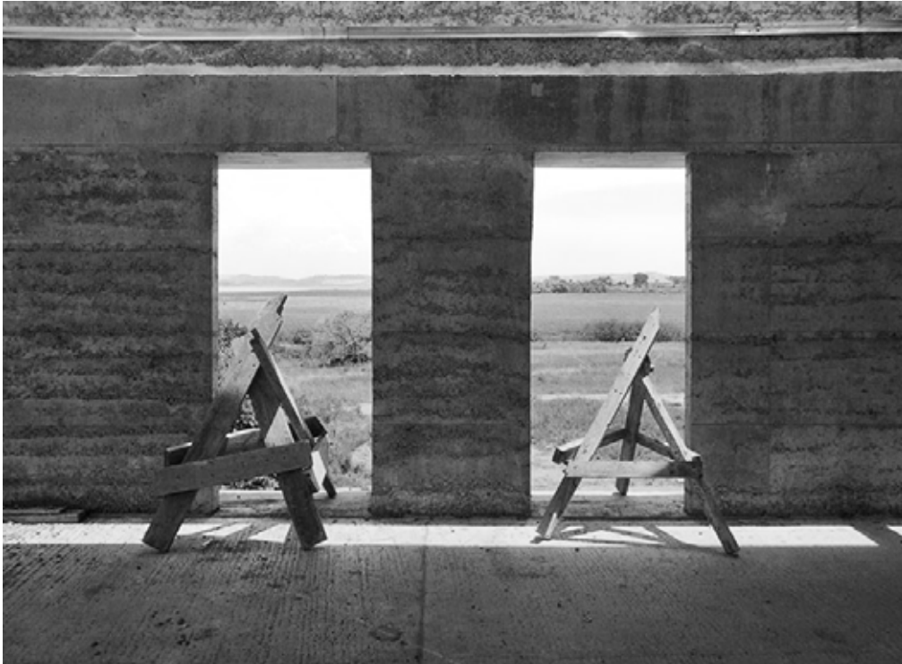
View to outside – rammed earth wall with reinforced ring anchor ill.[80]
