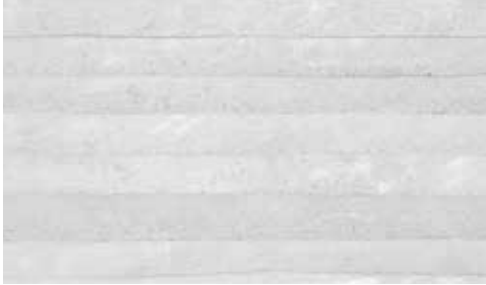
White lime plaster on rammed earth - walls
