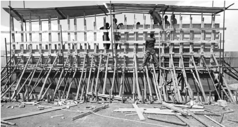
*Creating the formwork and rammed earth wall ill.[81]
