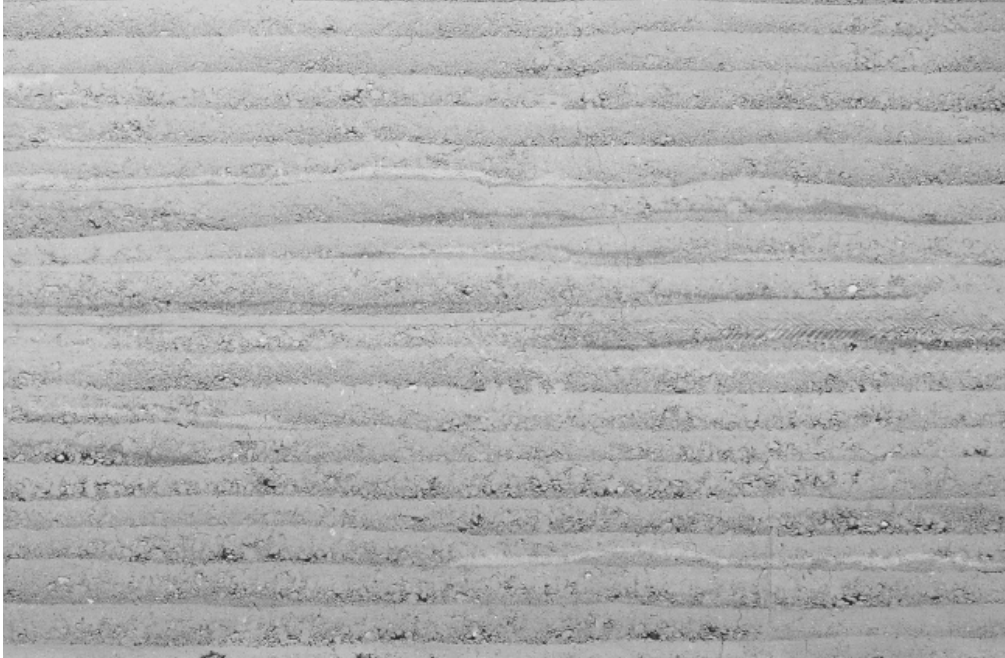
Texture of rammed earth wall ill.[49]
