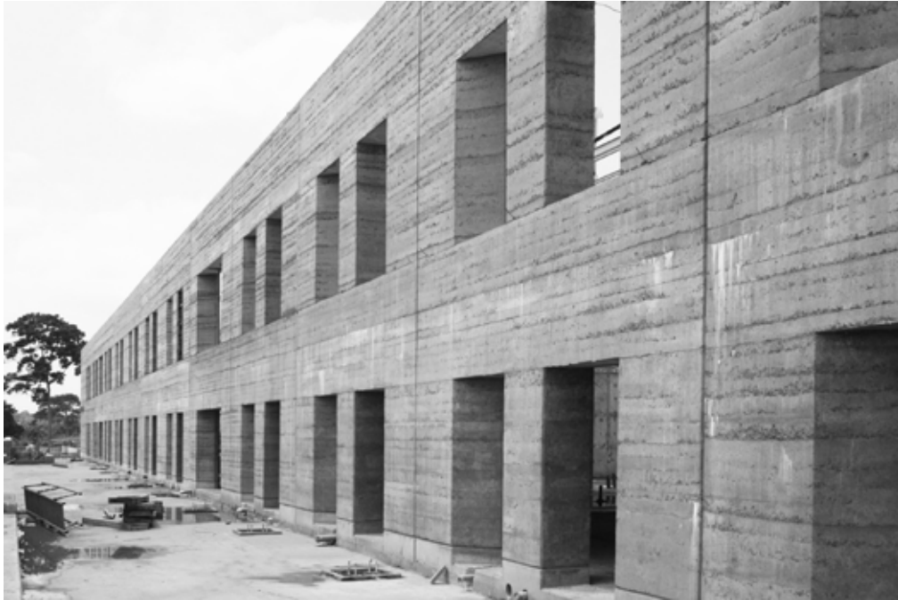
Rammed earth wall and the rhythm of the openings create atmosphere ill.[78]
