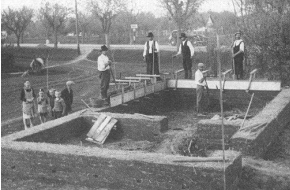
Construct the rammed earth wall requires the family and a brigade ill.[48]
