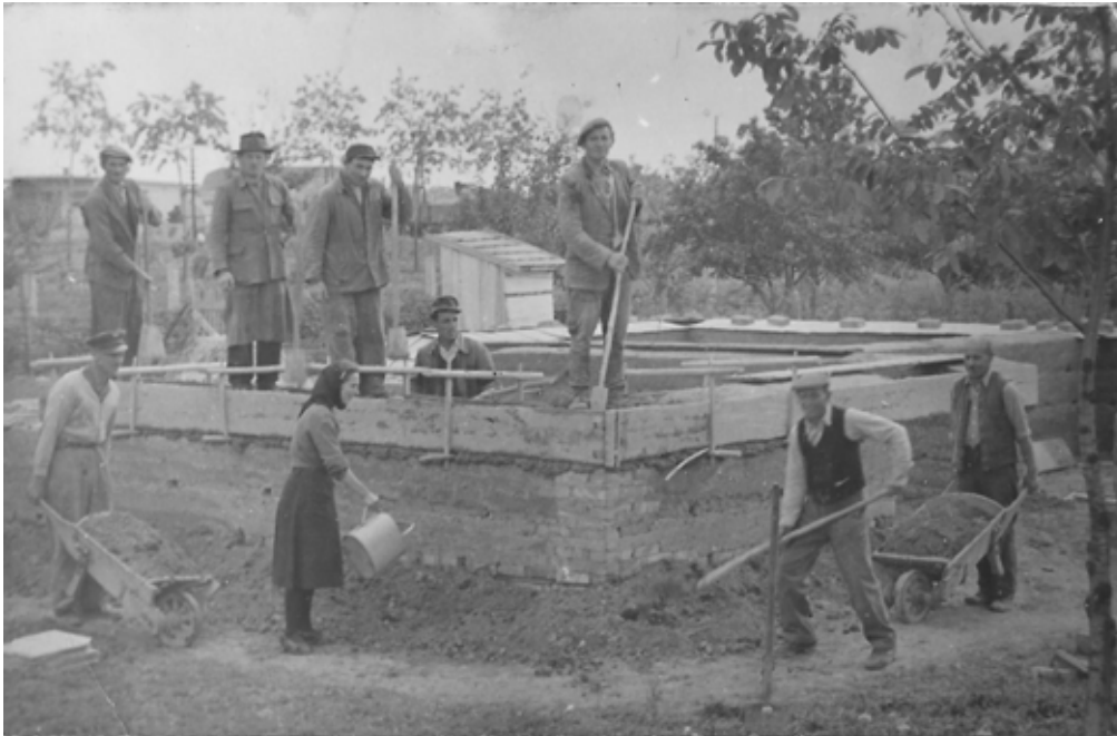
Construct a rammed earth wall in Kóny, HUN ill.[50]
