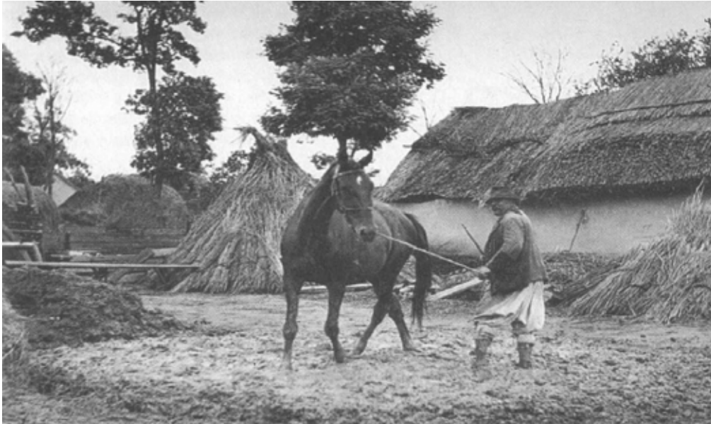
The earth is compressed by horse-power ill.[46]
