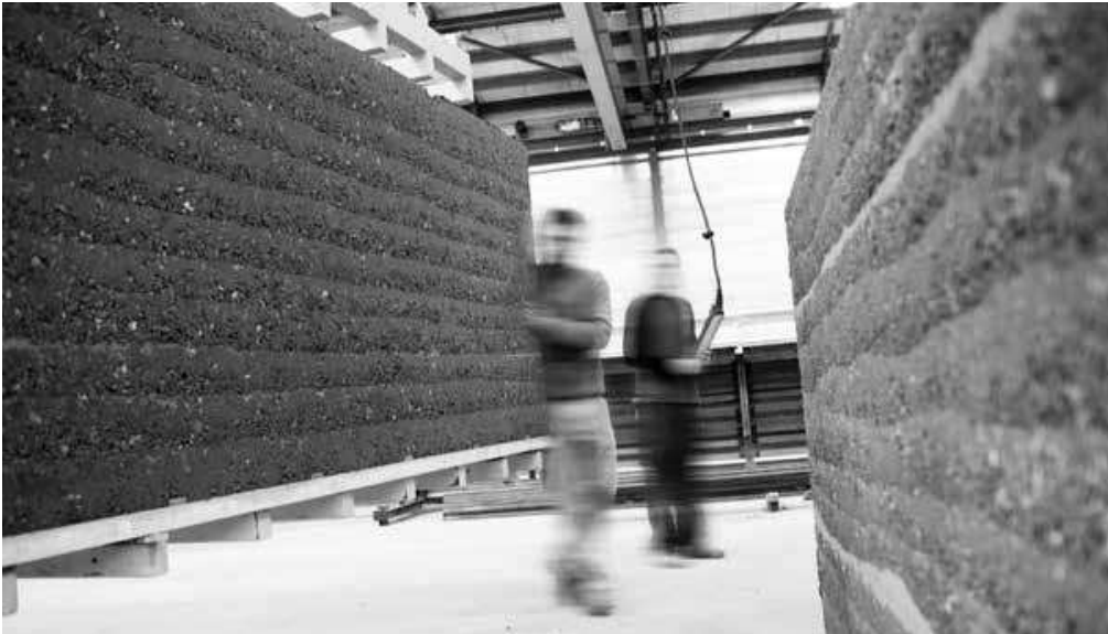
Fabrication of a rammed earth wall in a factory ill.[70]
