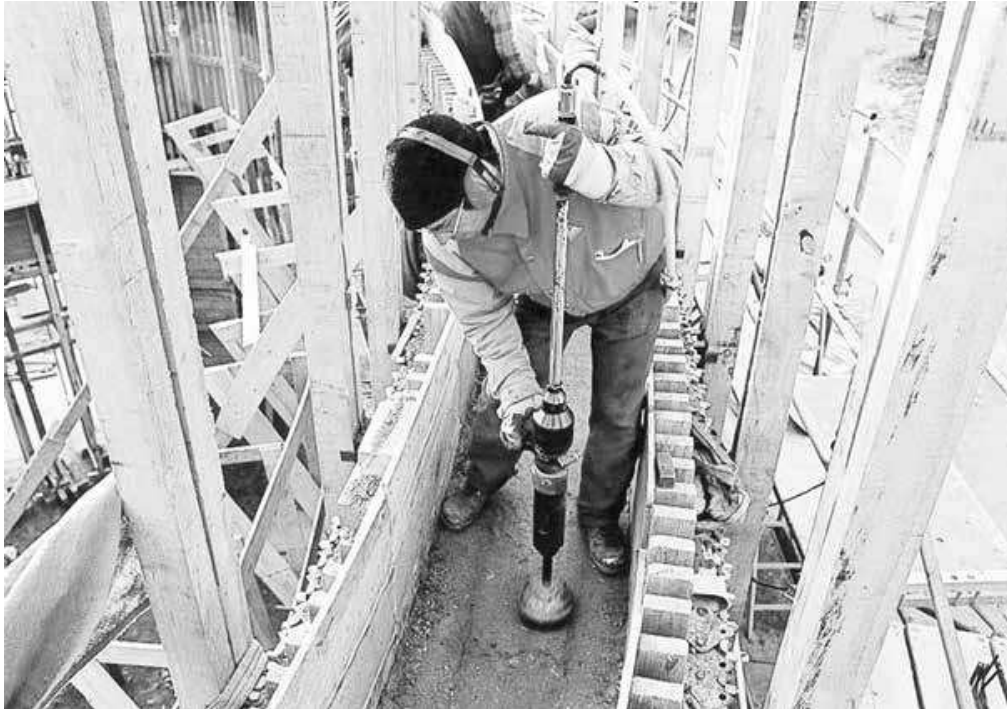
Fabrication of a rammed earth wall on site ill.[69]
