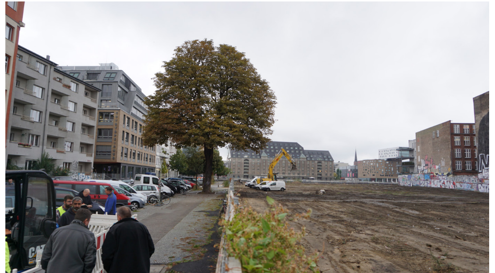
Fig. 41 street view Cuvystraße
