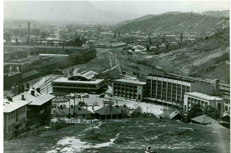
Fig 80. View of the Main Railway station and northern side of barracks
