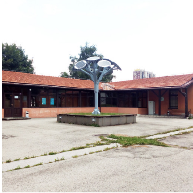
Fig 59. Lab and Solar Tree
