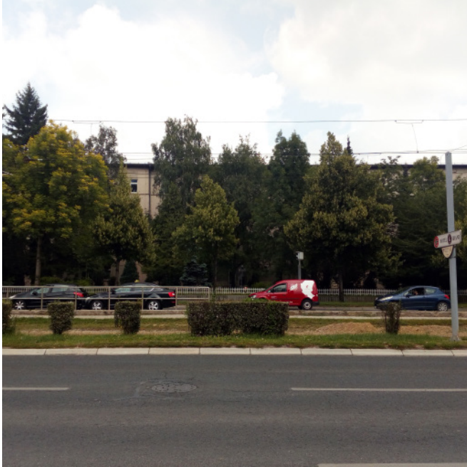
Fig 71. View From Main Street
