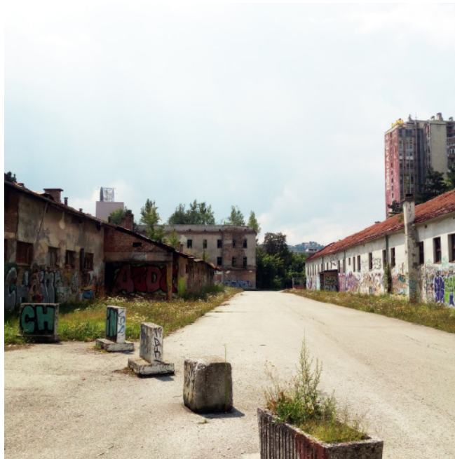
Fig 64. Damaged West Side
