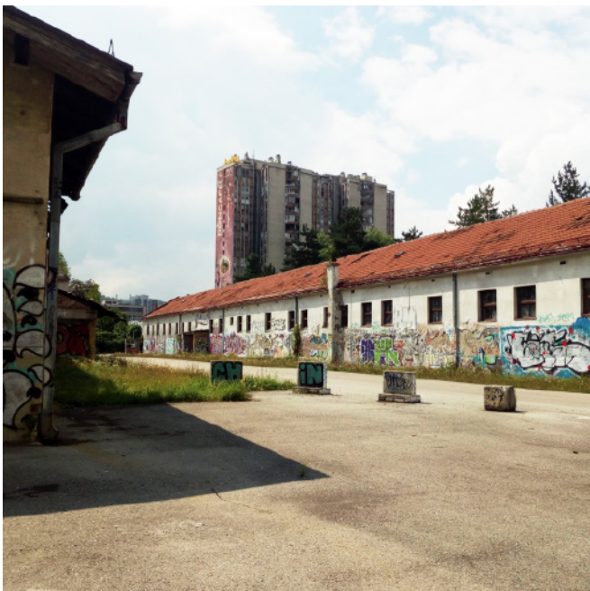
Fig 65. Damaged West Side
