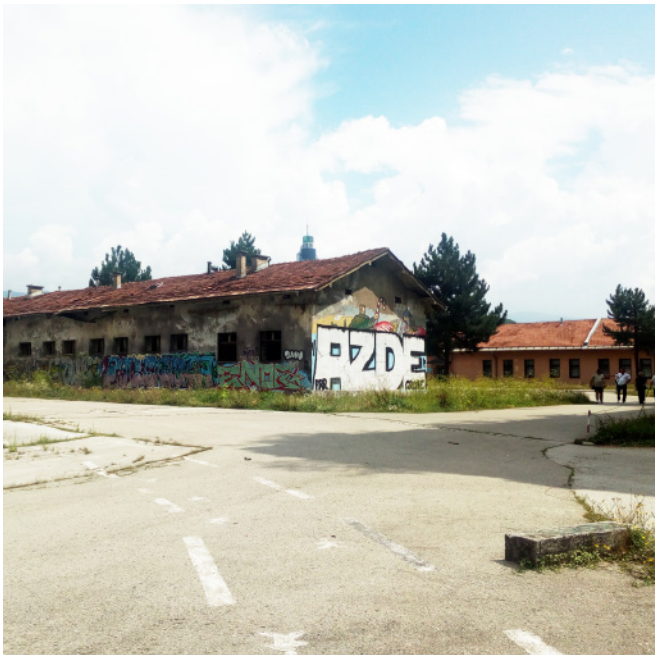
Fig 63. Damaged West Side
