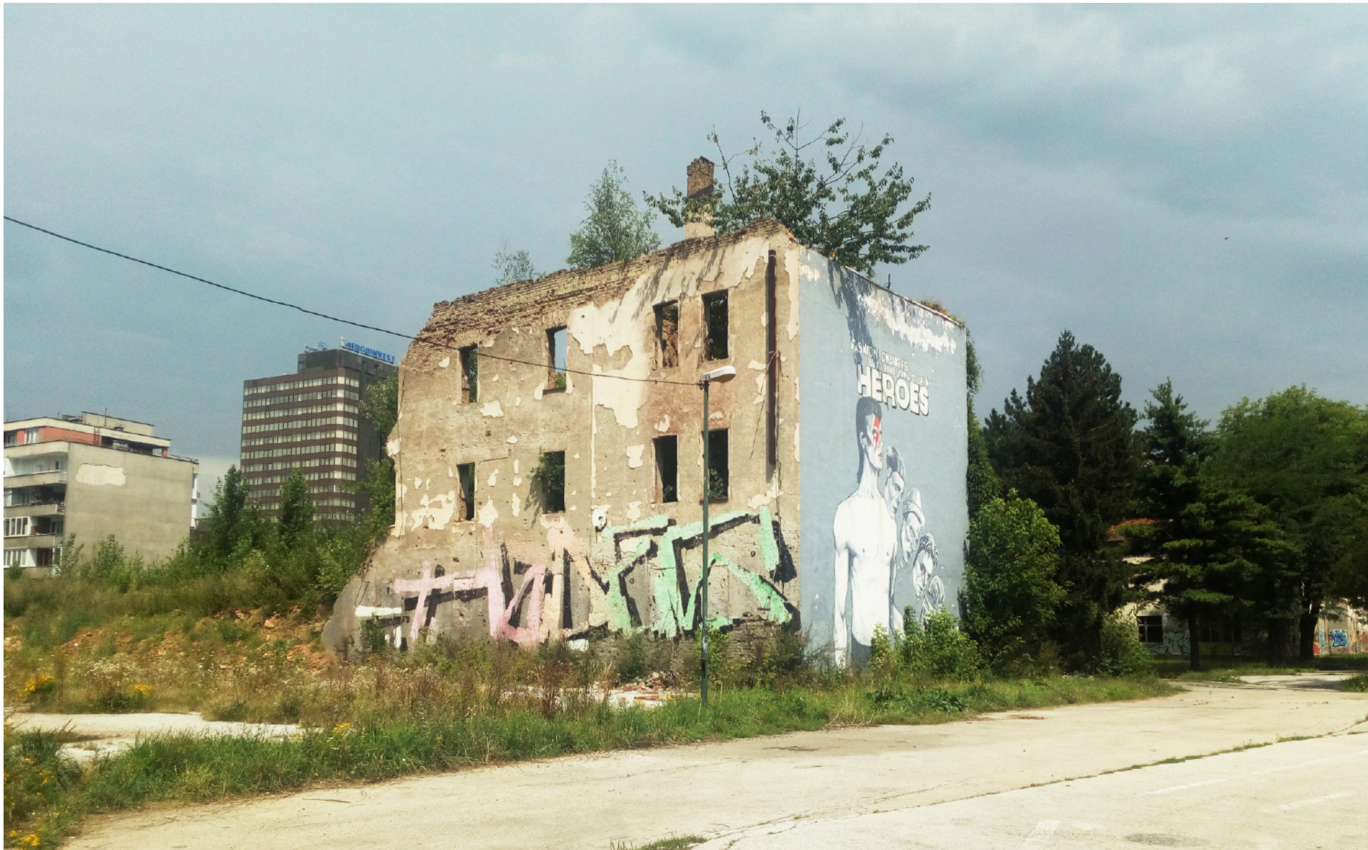
Fig 26. David Bowie Mural on site drawn on one of the destroyed buildings
