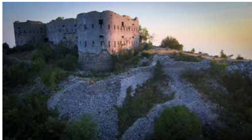
Fig. 179: Curve in front of the northern wing of Fort Kosmač, 2020 (The embankments collapsed) Credits: Ivan Varatnica
