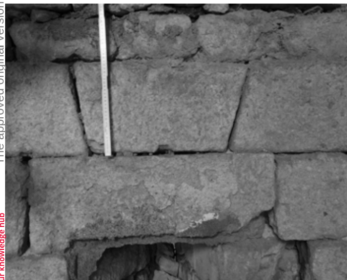
Fig. 78: Stone layers of the eastern barracks wall (Regular stone layer was made out of 25cm high stone blocks at wall faces. Inner faces were plastered with lime plaster) Credits: Ivan Vratnica
