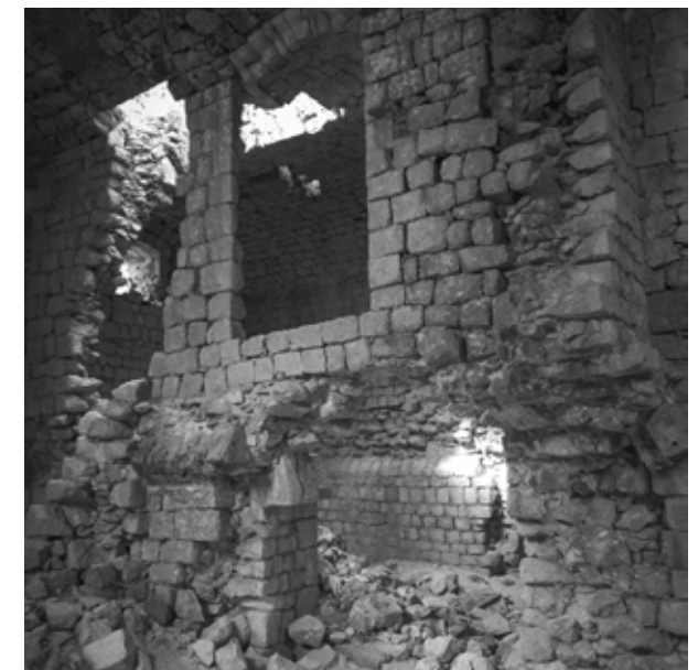
Fig. 122 (top right): Interior of the barracks Fort Kosmač, 2010 (Position of the chimney in the kitchen (16) that collapsed, critically weakening the bearing wall, making it deteriorate more over time) Credits: Radojica Pavičević
