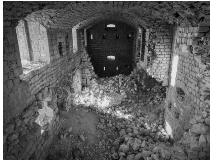
Fig. 195: Fort Kosmač, 2020 (Entrance to the barracks and the northern wing middle wall, missing its lower part) Credits: Ivan Vratnica
