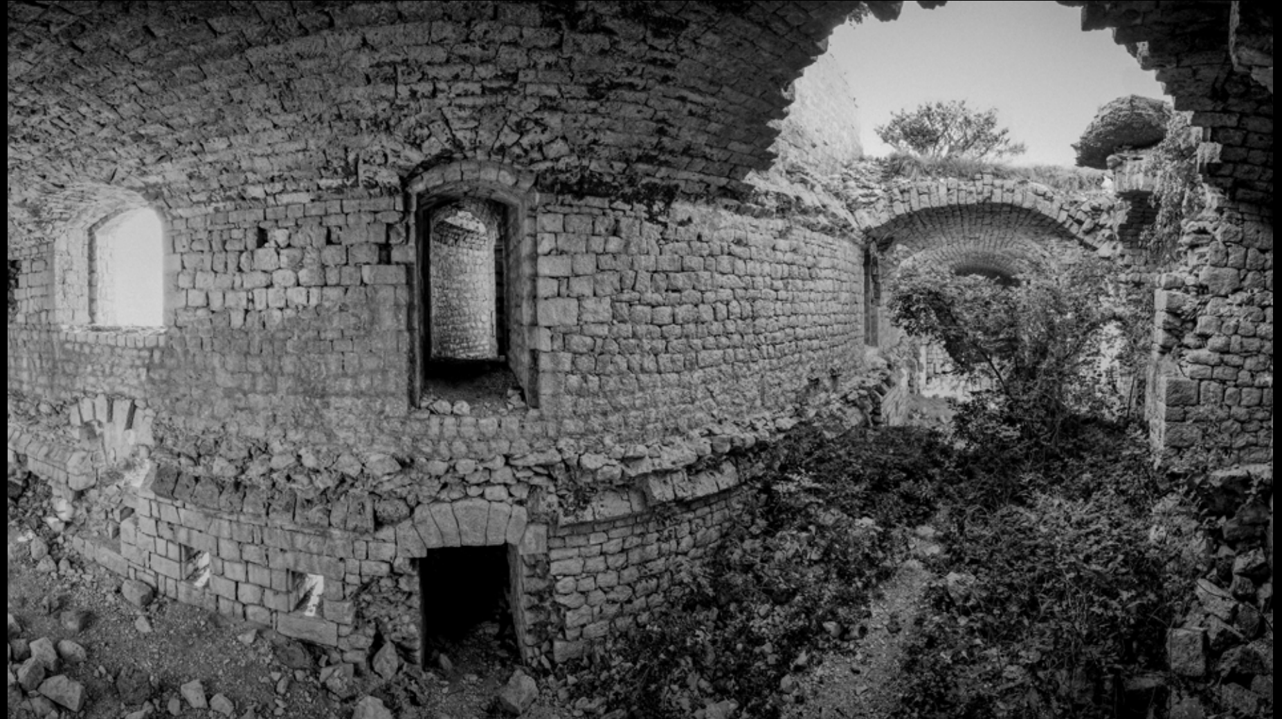
Fig. 204: Fort Kosmač, 2020 Middle of the barracks main tract (the vaults above collapsed and piled up in the round floor, filling it up, pushing against the outer wall) Credits: Ivan Vratnica
