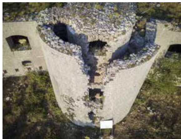
Fig. 192: Fort Kosmač, 2020 (Outer wall of the western wing almost split in two as the window arches collapsed) Credits: Ivan Vratnica
