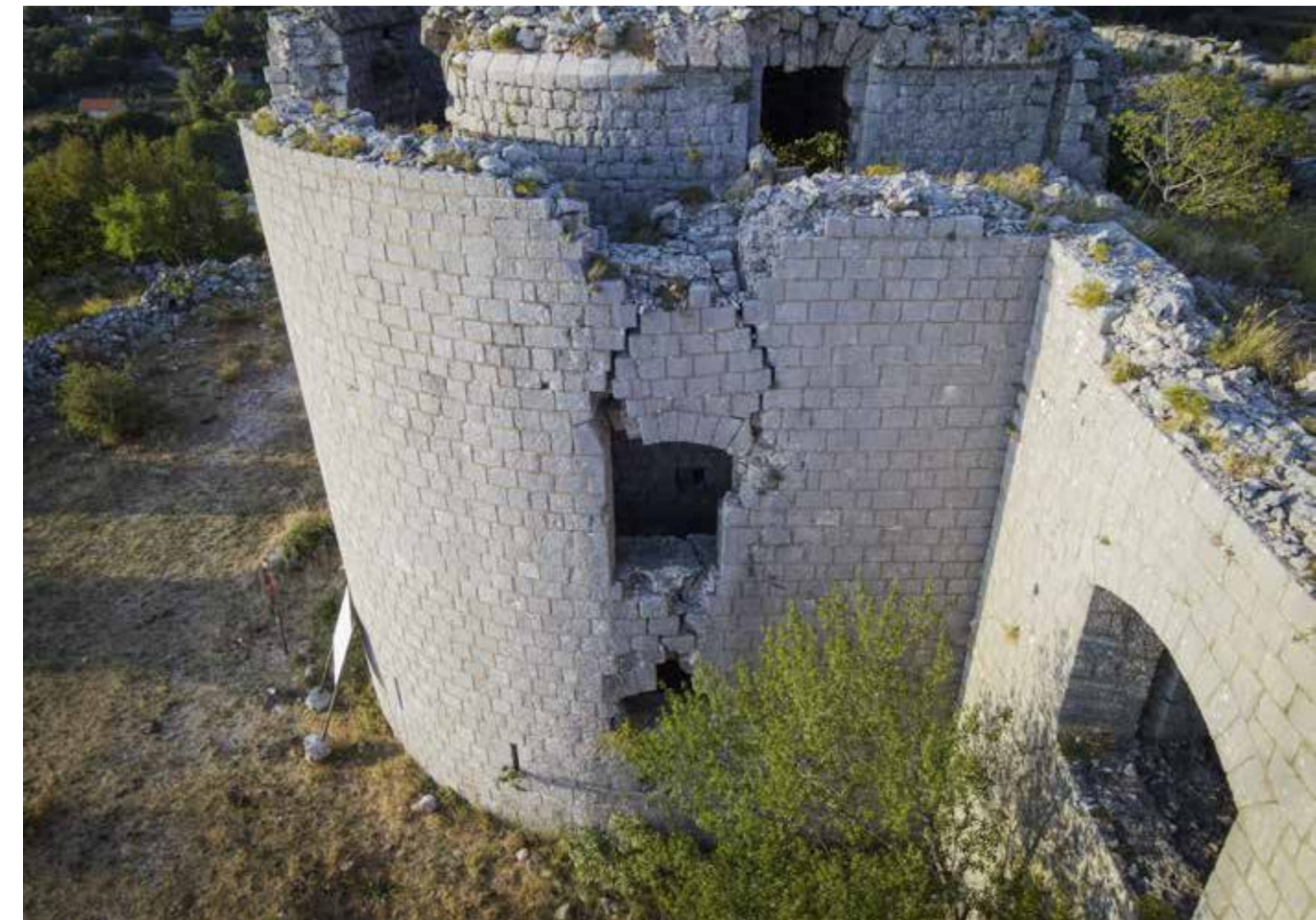
Fig. 193: Fort Kosmač, 2020 (The side window arch loosened as the outer wall of the wing tilted outwards) Credits: Ivan Vratnica
