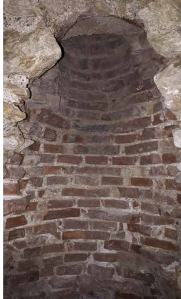
Fig. 74: Remaining of a chimney in the ground floor, 2019 (Chimneys are the few elements where bricks were used instead of stones) Credits: Ivan Vratnica
