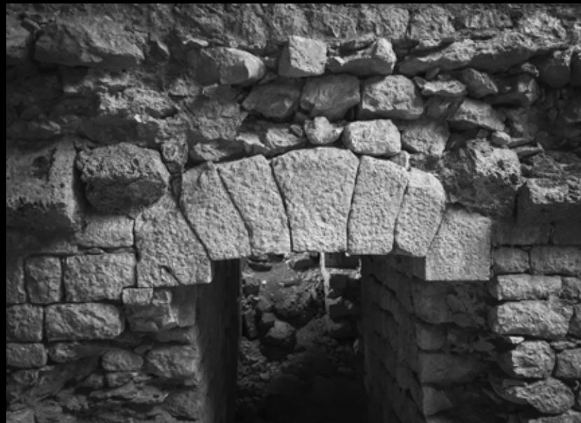
Fig. 143: Stone arch construction of the door to the passage (26) Fort Kosmač, 2019 (The vault construction above collapsed leaving the arch visible) Credits: Ivan Vratnica
