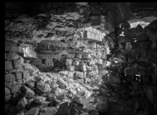
Fig. 135 (top left): South-eastern wing Fort Kosmač, 2019 (Provisions storage (21) in the ground floor and crew quarters (30, 31) above. The only remaining part of the vault between ground and the first floor) Credits: Ivan Vratnica
