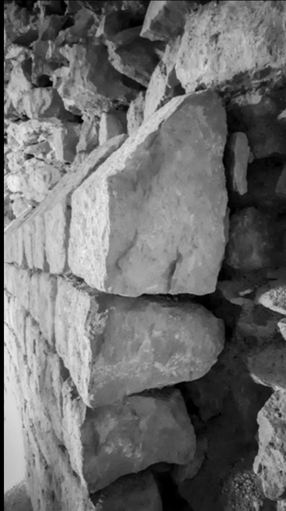
Fig. 203: Fort Kosmač, 2020 Slanted stone layer on which the vaults were leaned Credits: Ivan Vratnica
