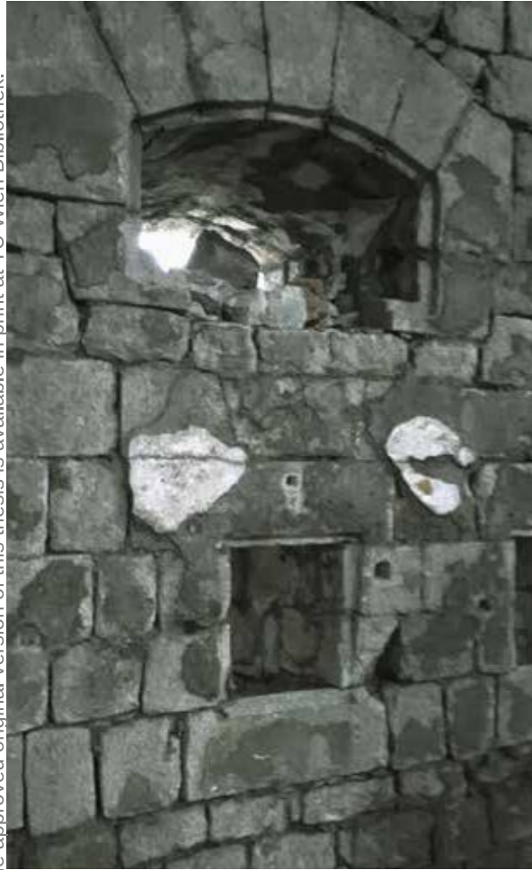
Fig. 73: Wall surface inside the ground floor, 2019 (The parts of the cement and white plaster are still visible on some spots, as well as the carvings around the window frames where the wooden frames with casements were attached to the stone wall with metal nails)
