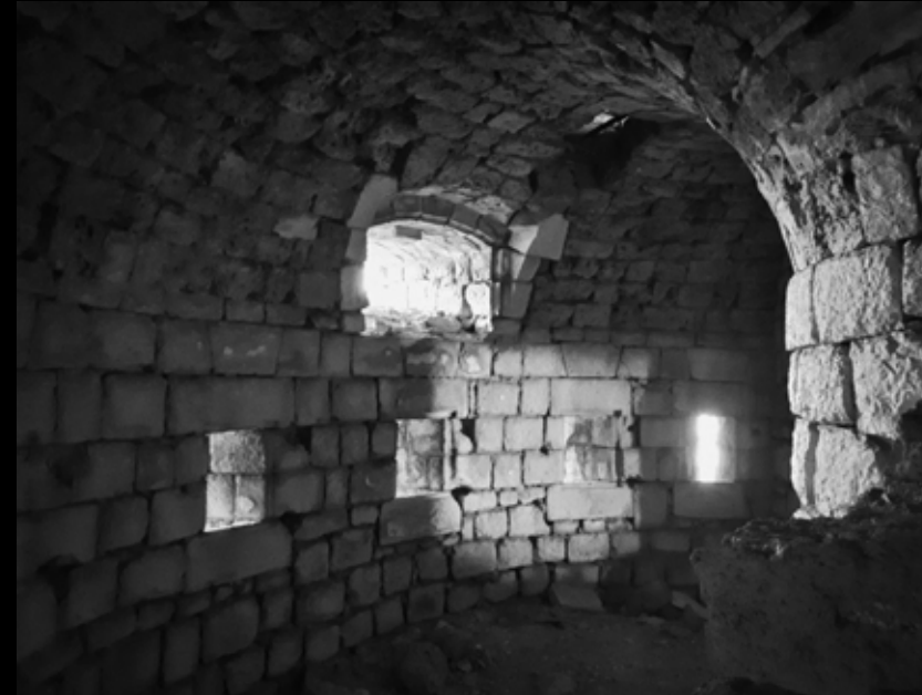
Fig. 144: The provision storage (23) in the south-eastern wing Fort Kosmač, 2019 (The half circular vault construction still present) Credits: Ivan Vratnica
