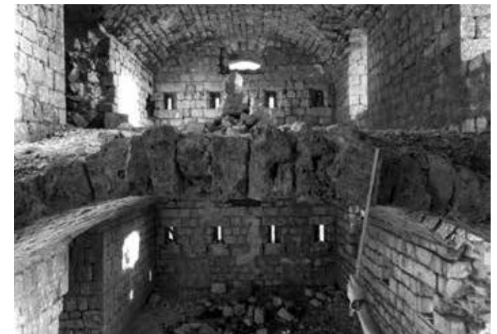
Fig. 80: The last remaining part of the first floor vault (The vault is 30cm thick made of "Siga" stone) Credits: Ivan Vratnica
