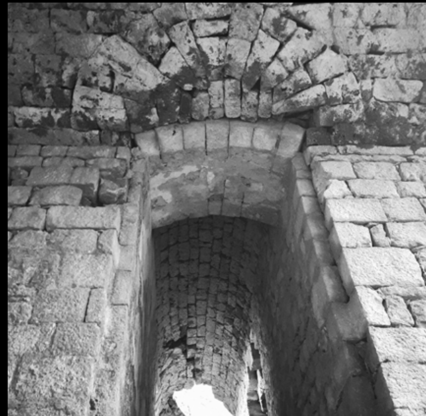
Fig. 145: Stone arch construction of the door to the stairway (26) Fort Kosmač, 2019 (The vault construction of the door above is still visible compared to the previous photo) Credits: Ivan Vratnica
