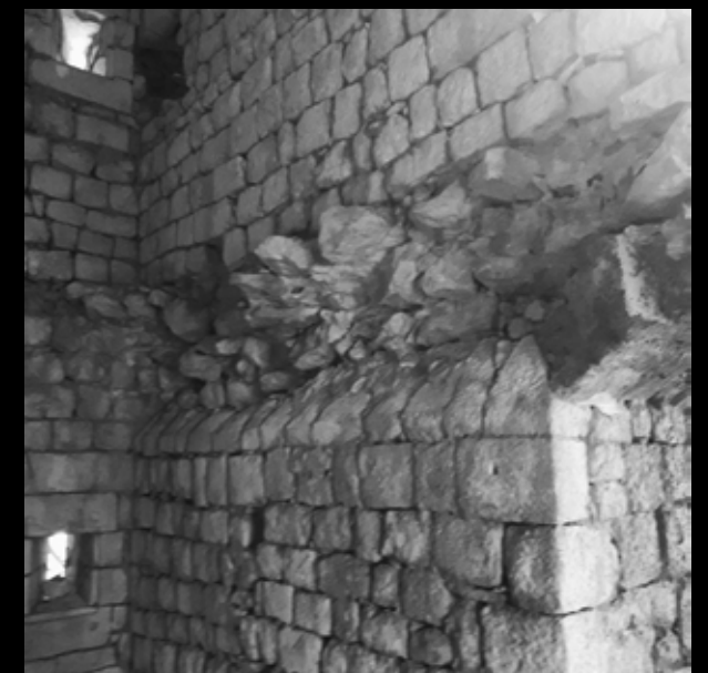
Fig. 137 (top right): Southern part of the main tract Fort Kosmač, 2019 (The biggest hole in the eastern wall in the corner of the crew quarters (18) and the provisions storage (22). Loopholes closed during the uprising 1869 ) Credits: Ivan Vratnica
