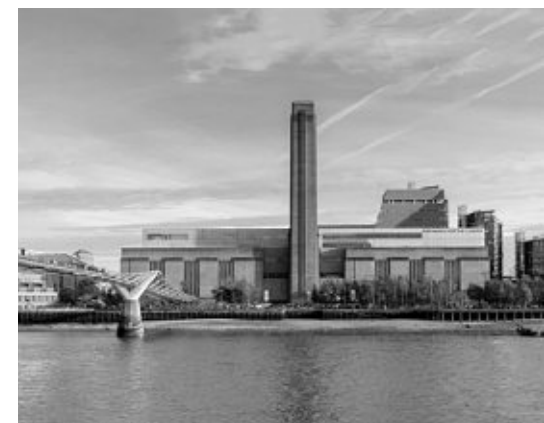
adaptive reuse city regeneration
