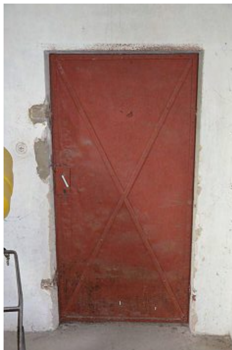
Abb. 136: Tür T-E2.1 in Wand W-E1.B, Mai 2020
