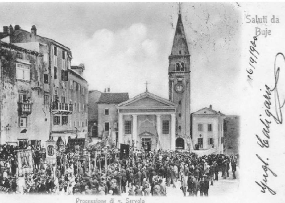
Figure 15, Former appearance of the Square of Liberty
