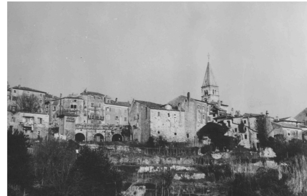
Figure 18, Former appearance of the substructure and Square of Liberty from the south
