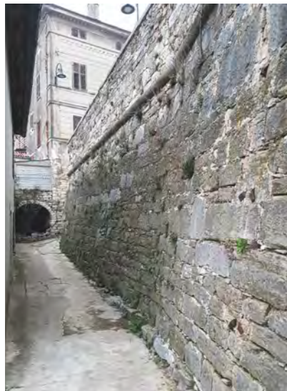
15_Passage to the old Structure
