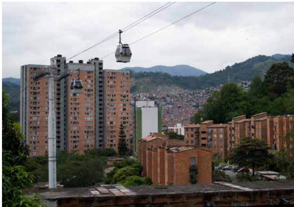
Fig 71. The Cable Car going from San Javier Metro Station towards the barrio Juan XXIII. [Photo taken by the author, 2017]
