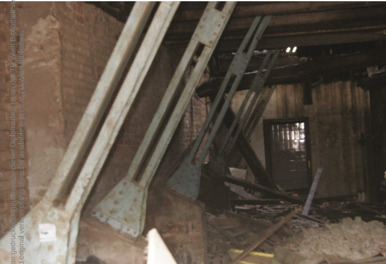
Fig. 67. View on the slanted support beams
