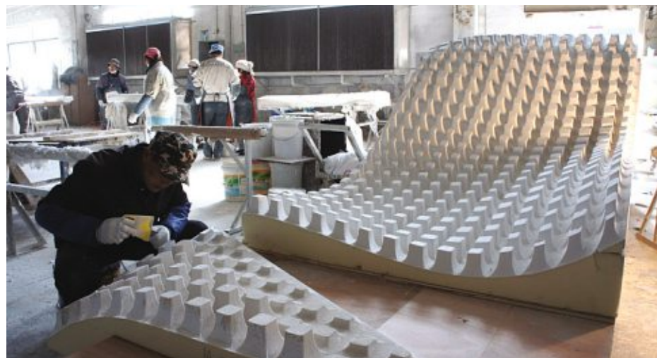
Fig. 89. Facade of the MaoHouse - production process
