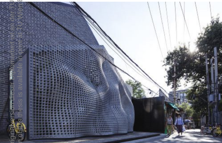
Fig. 87. Facade of the MaoHouse
