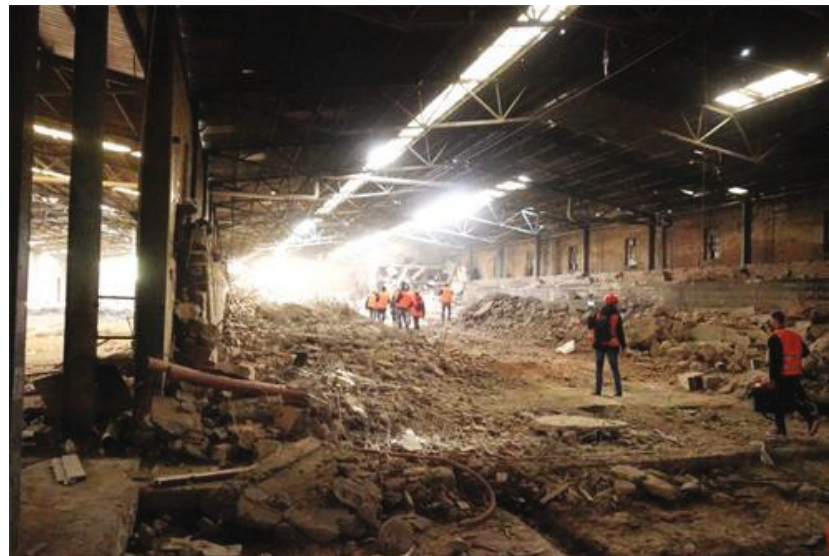
Fig. 47. Interior of the storage building, pictured rescue practice
