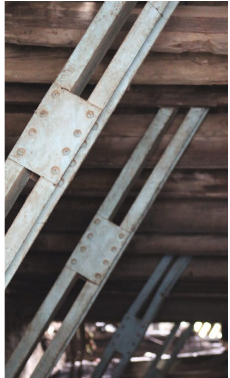
Fig. 68. View on the slanted support beams
