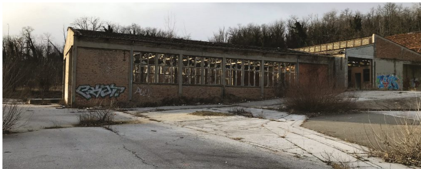
Fig. 48. Clay processing building
