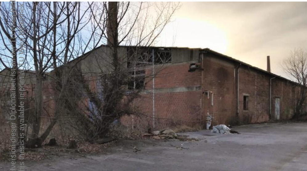
Fig. 46. Storage building adjacent to the brick factory
