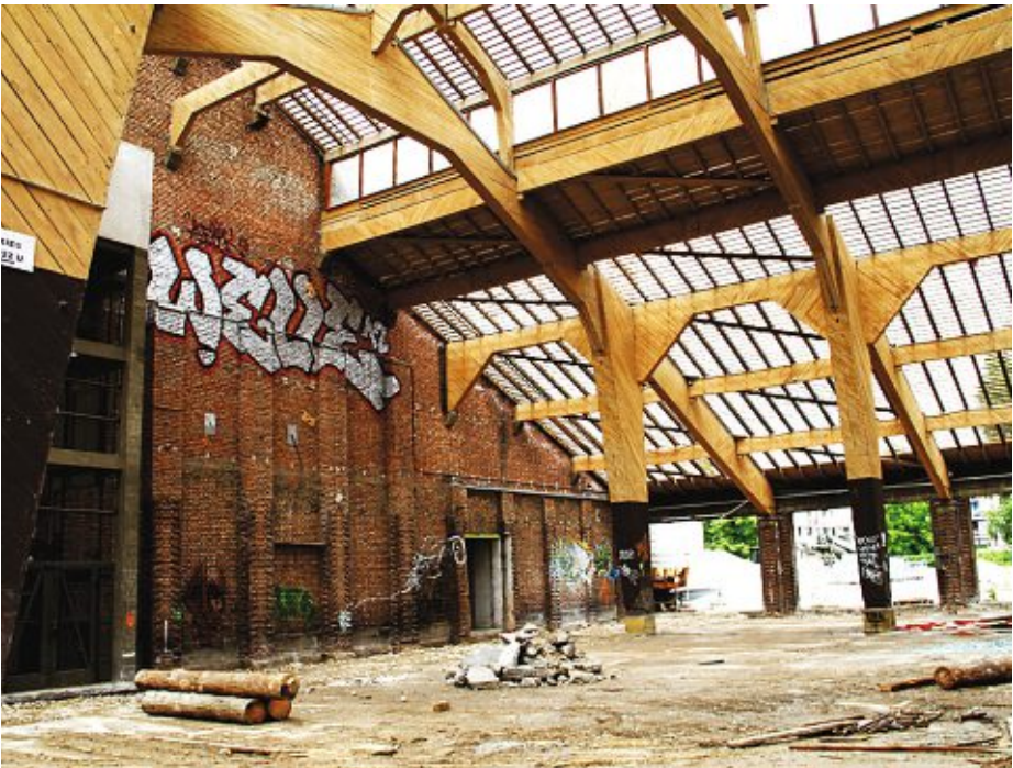
Fig. 33. (above) Panzerhalle interior before repurpose
