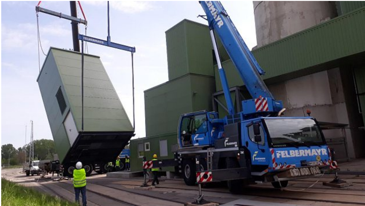
Figure 6-1: Erection of pilot unit in Wien Simmering
