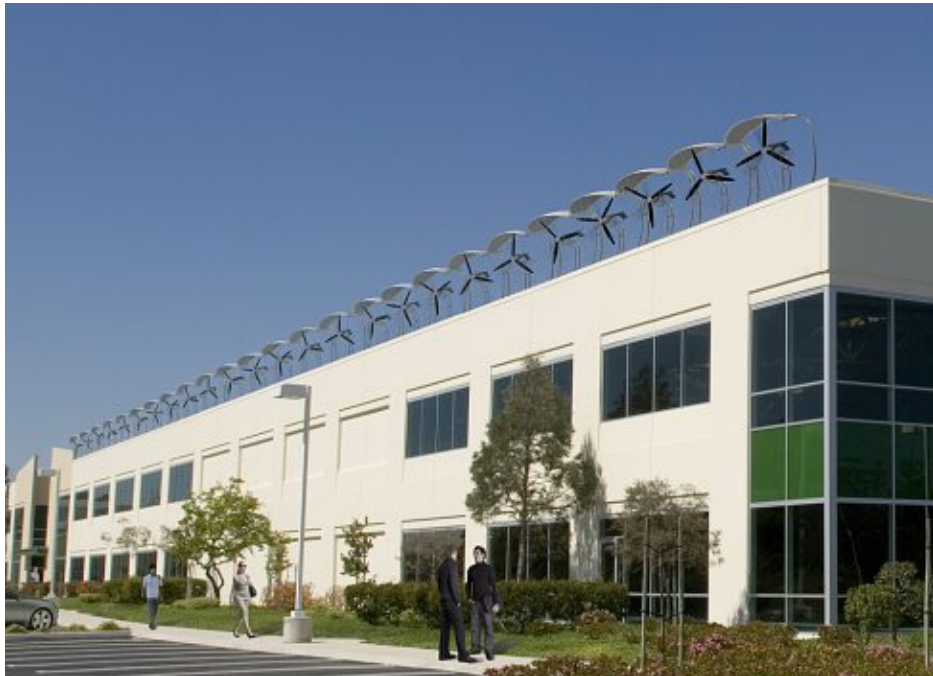
Figure 18 Project for small wind turbine integration on a rooftop (Source: Building-integrated wind turbines 2016)
