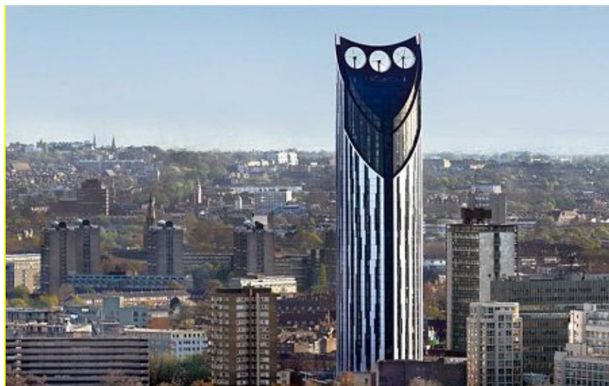
Figure 13 Strata Tower, London (source:Teh 2016)
