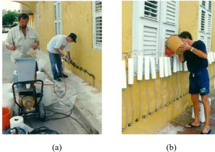
Figure 5.12 (a) Wall treatment using pressure (injection), and (b) wall treatment using only hydrostatic (Impregnation)
