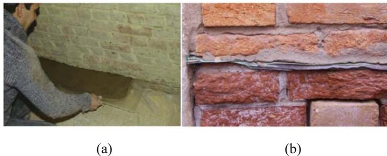
Figure 5.11 (a) Mechanical interruption Italy (Universita Ca'Foscari Venezia), and (b) Mechanical Interruption in Belgium (BBRI) (source: EMERISDA 2014)
