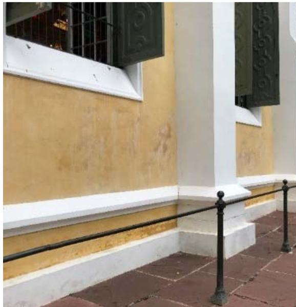
Figure 3.8 Signs of post-retrofit moisture problems on the middle and lower parts of the walls (photo taken in 2017) (source: Pinich 2018)
