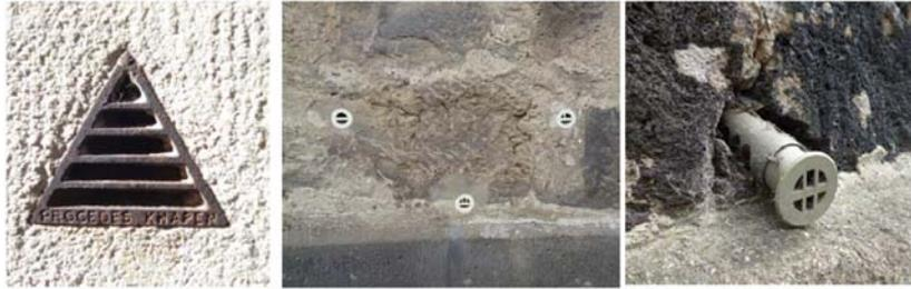
Figure 5.7 Different types of Knapen siphons in wall
