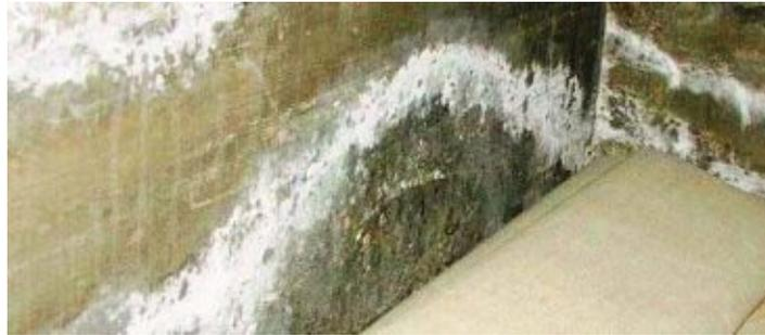
Figure 4.1 Efflorescence on the wall surface
