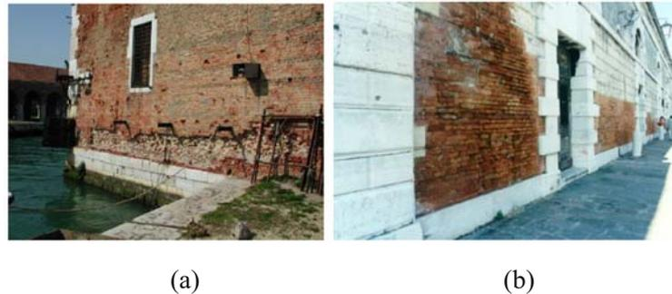
Figure 5.9 Horizontal courses of low-porosity stones brick were used at the base of the walls in order to limit the water capillary rise in two affected buildings in Venice; (a) Alberaria Tower, and (b) Salt Emporium (source: EMERISDA 2014)
