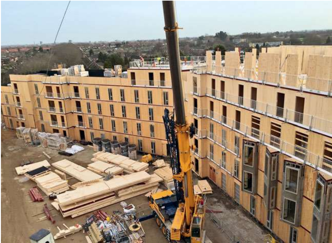
Figure 3-4: Building site assembly using 2D CLT panels [2, p. 96]
