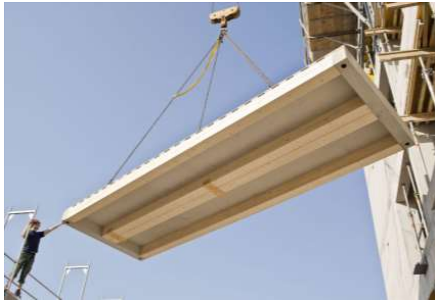
Figure 4-7: Prefabricated TCC floor element, LCT-One Tower [31, p. 4]
