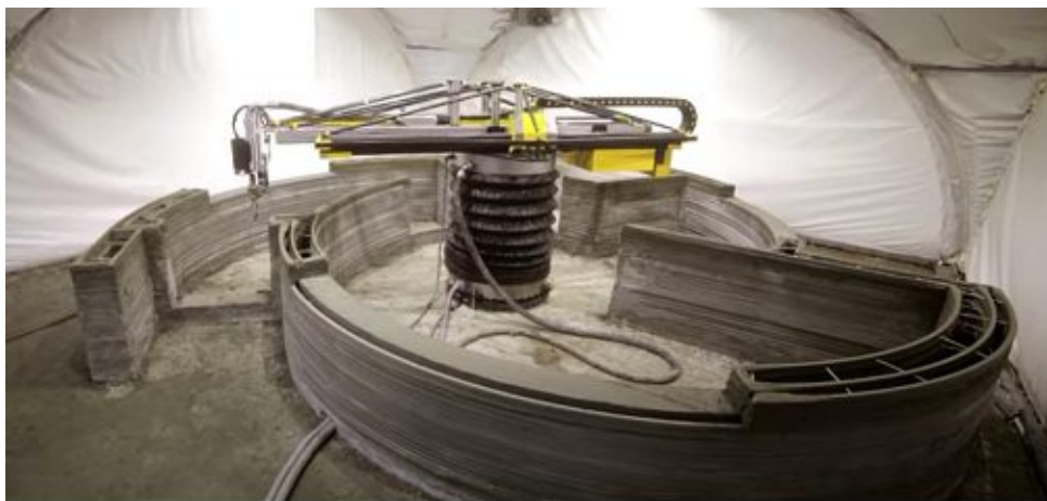
Figure 18- First 3d printed house (Quartz, 2017)
