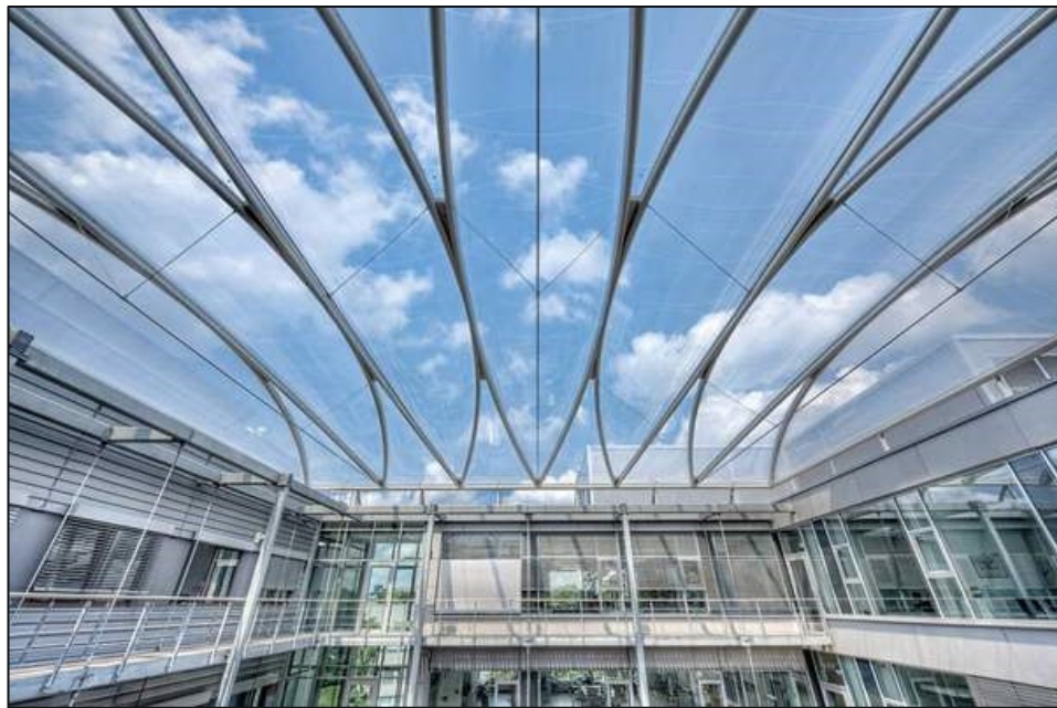
Figure 25: ETFE cushion roof, DWI – Leibniz Institute for Interactive Materials, Aachen, Germany (website: airsculpt.com ) 15
