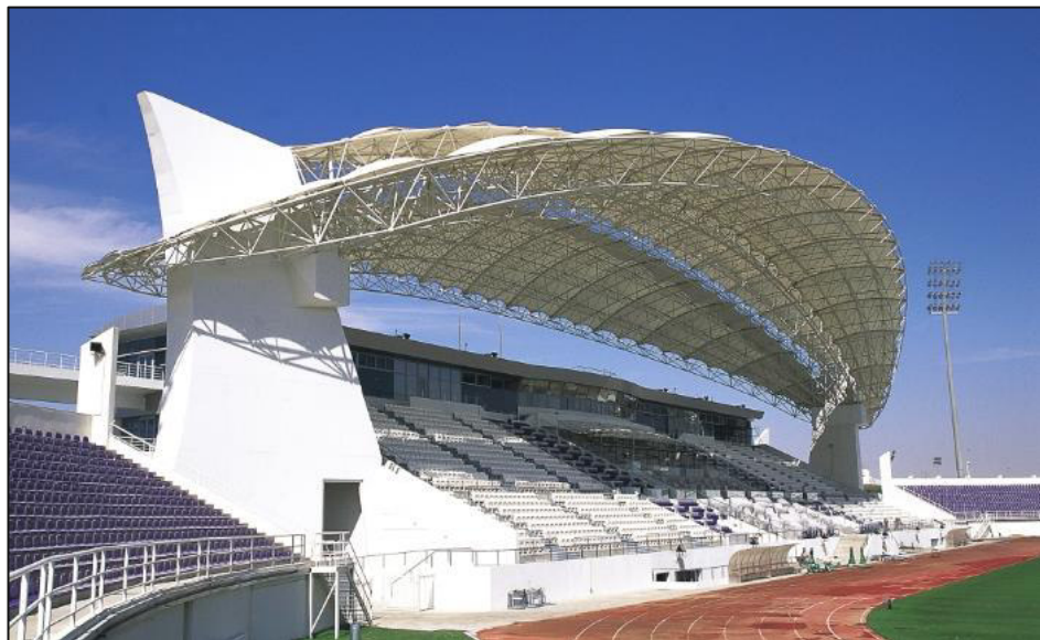
Figure 17: Grandstand Roof, Sheikh Khalifa Bin Zayed International Stadium, Al Ain, U.A.E. (website www.structurae.net ) 9
