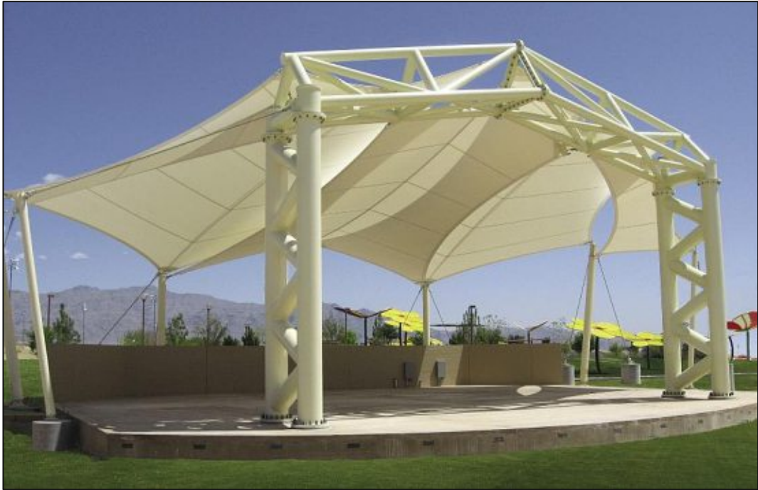
Figure 23: Massive steel front frame of a stage roofing (website www.archiexpo.com ) 13
