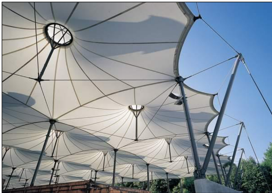
Figure 26: Collapsed former roof of car pool, office for waste management, Munich, Germany (website: DETAIL inspiration: inspiration.detail.de ) 16
