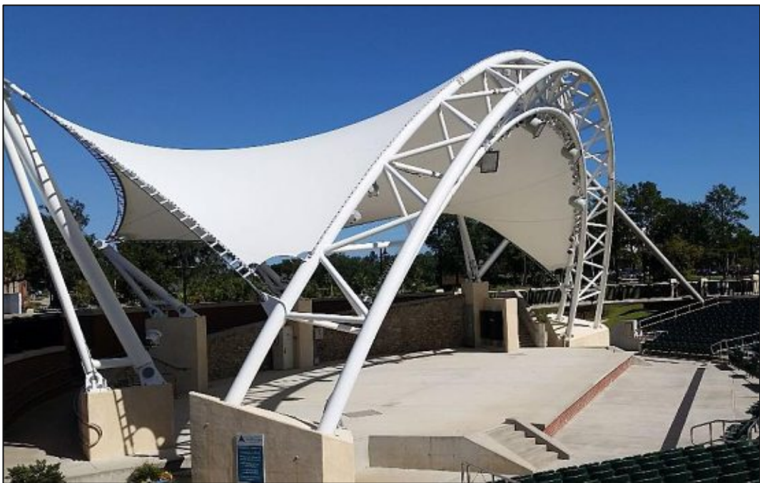
Figure 24: Massive steelwork of a stage roofing (website www.tallyishome.com ) 14
