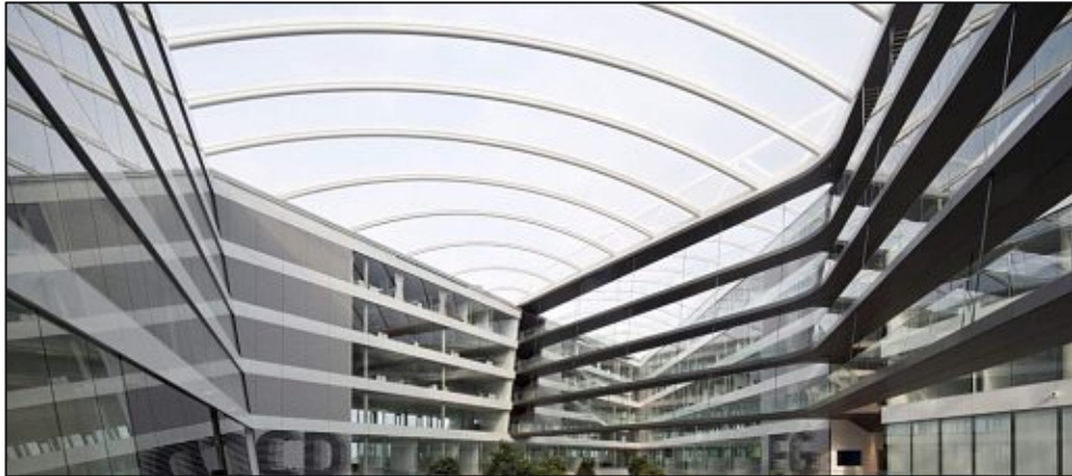
Figure 19: Long arched ETFE cushion roof without interconnecting members Adidas Laces, Herzogenaurach, Germany (website: architecturelist.com ) 11
