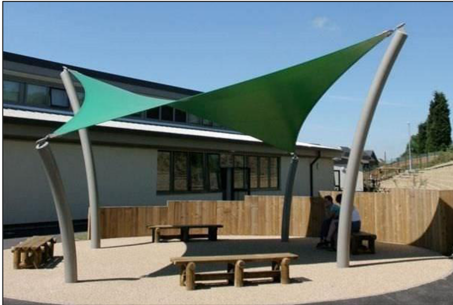
Figure 12: Hypar with four columns under bending (website areatenda.com ) 6
