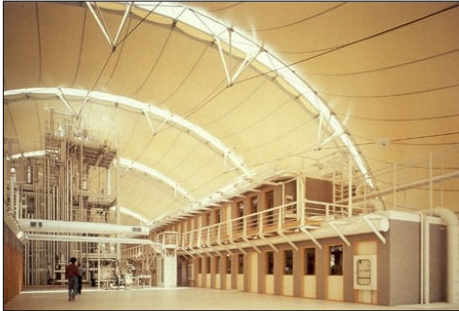
Figure 28: Roof over the Chemical Research Centre, Venafro, Italy – Internal view with the arches inter-connecting cables (website: samynandpartners.com ) 17
