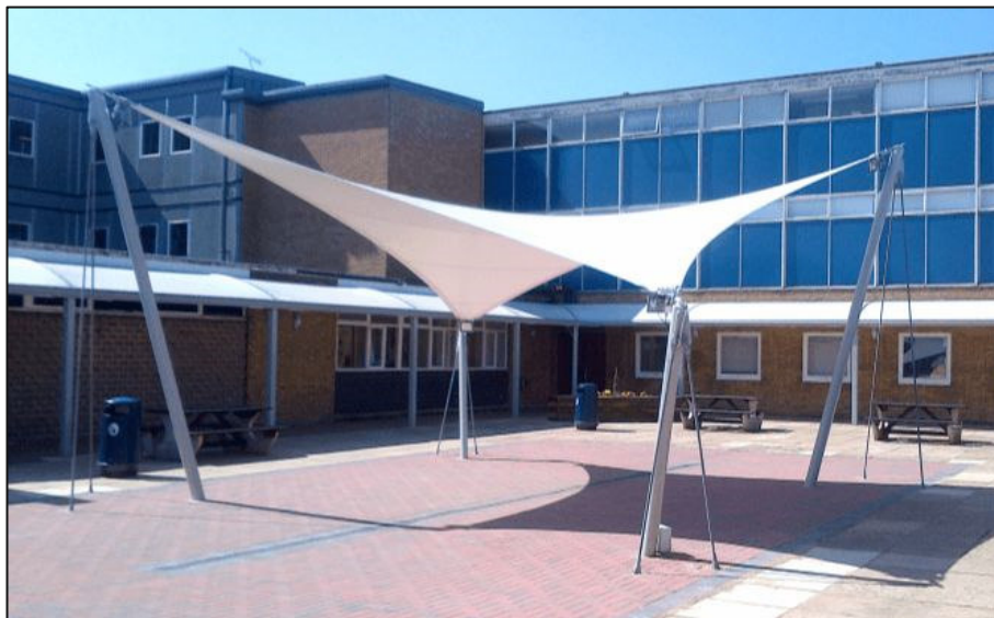
Figure 11: Typical hyper – Axial forces type – Slender (website www.jjcarter.com ) 5
