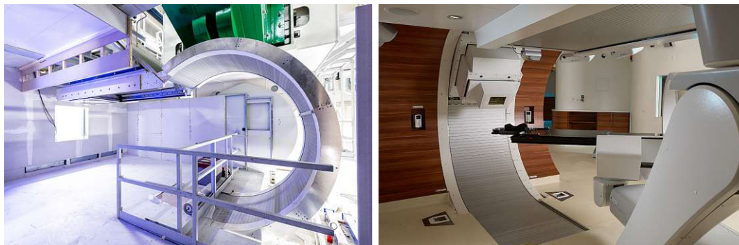
Figure 2.16: Two pictures of the IR4 to show the implementation of the rotational angle of the beam nozzle around the patient [67]. On picture (a) IR4 is seen during the construction phase, with the last bending magnet in green above the roller shutter. In (b) the finished IR4 with the installed beam nozzle in the roller shutter and the treatment table, held by the patient positioning system is seen.
