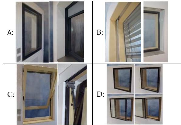
Fig. 4 – Opening/operation schemes of prototype A – D.
