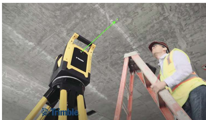
Abb. 3.26: Einmessen mittels Robotic Total Station von Trimble [162]
