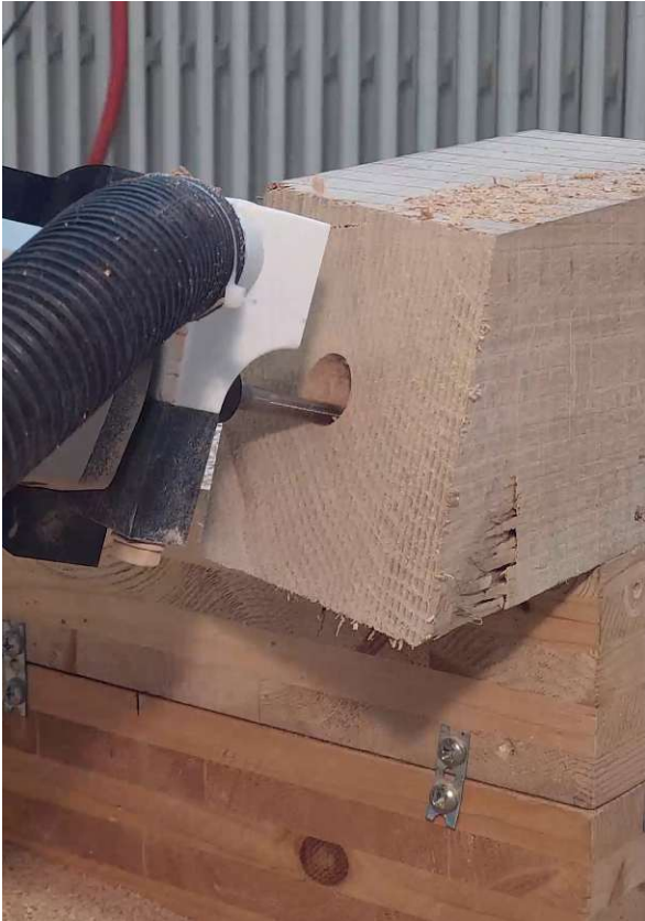
Figure: 69 – KT2 - Drilling Center.
