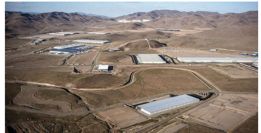
Abb. 60 Tahoe Reno Industrial Center
