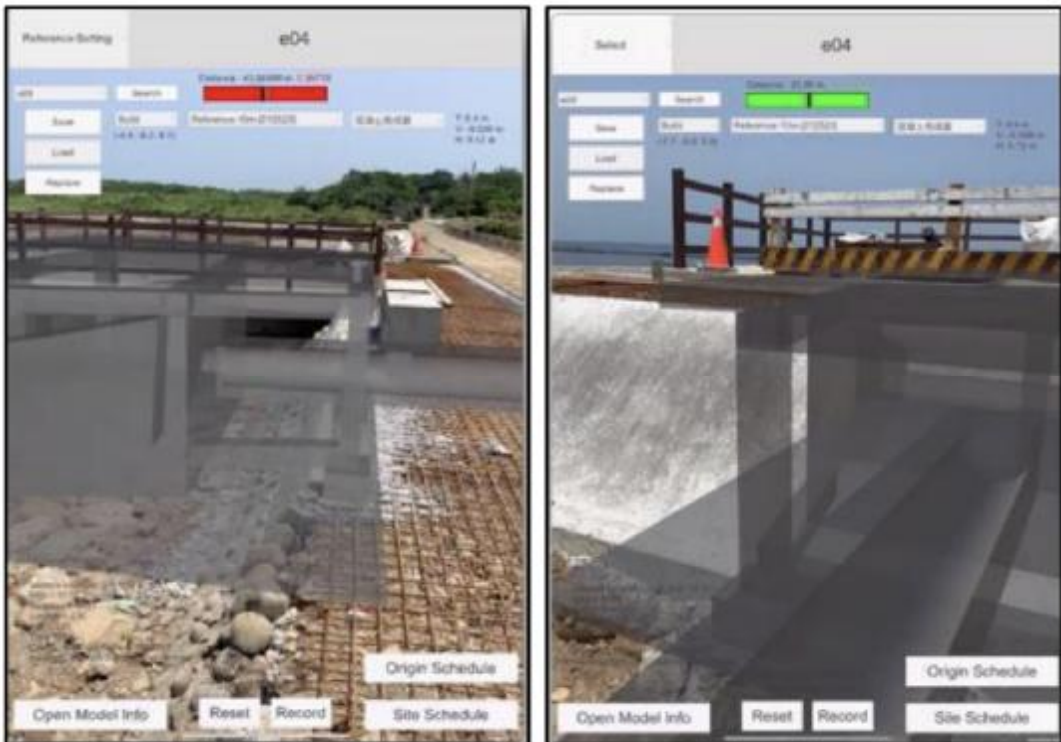
Fig. 15: Excavation depth confirmation on the construction site
