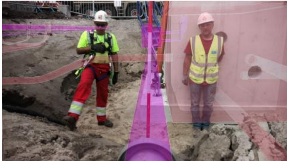
Fig. 31: The installation of the prefabricated concrete chambers (2)
