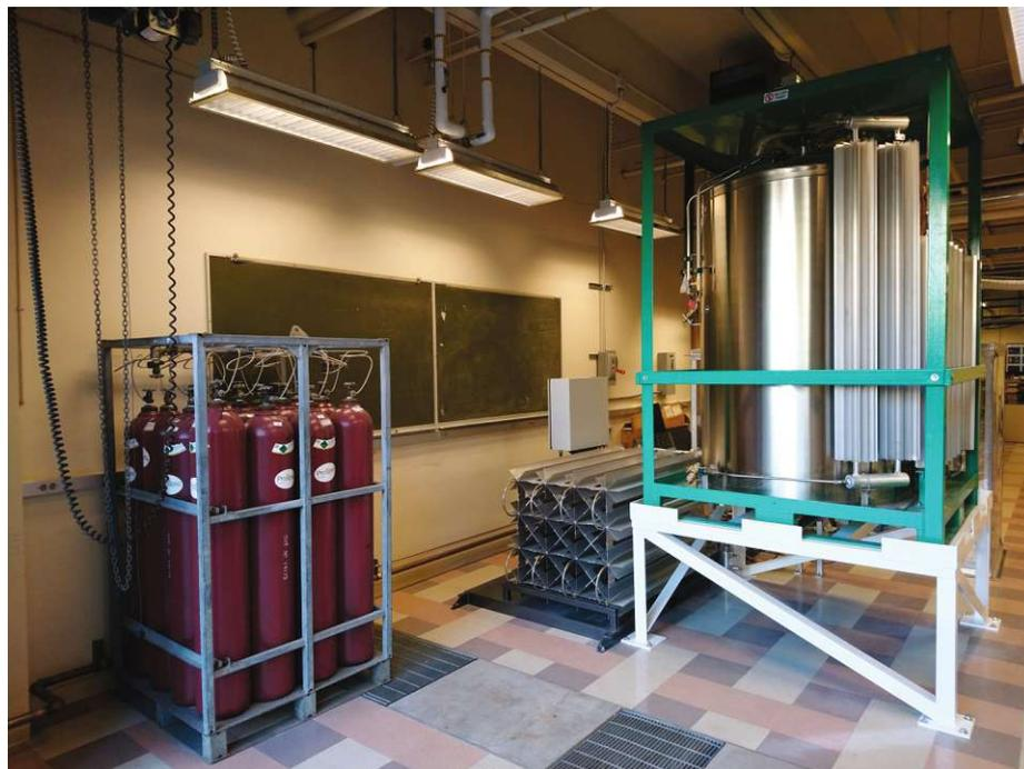
Figure B.11: Nitrogen Supply System - Portable tank on stand (right), vaporizer and control station assembly (center), and high pressure cylinder pack (left).
