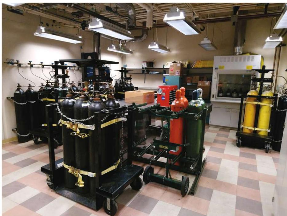
Figure B.10: Nitrogen Supply System - Cylinder carts carrying a manifold of pressurized gas cylinders providing various gases to the HPCEF.
