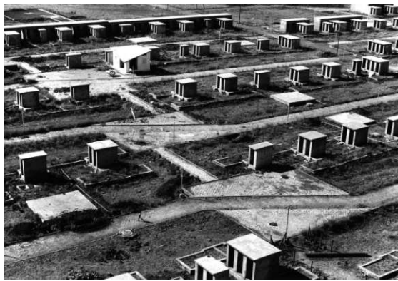
(a) Initial view with plinth and sanitary room
