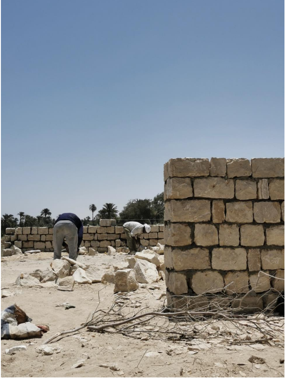
fig. 71. dabsch , Mansour's construction site
