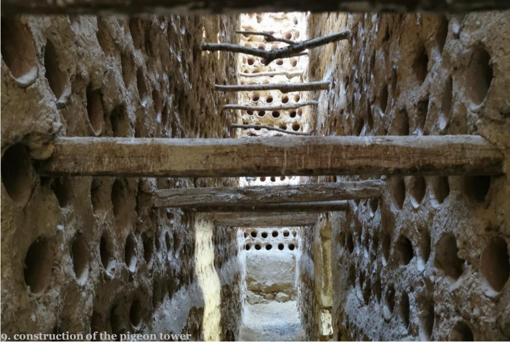
fig. 169. construction of the pigeon tower
