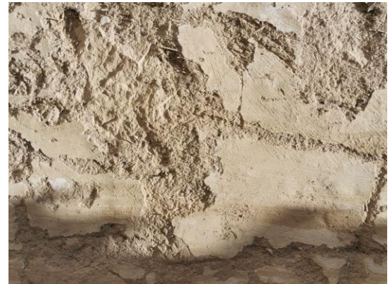
fig. 57. cement plastering of the fallah house
