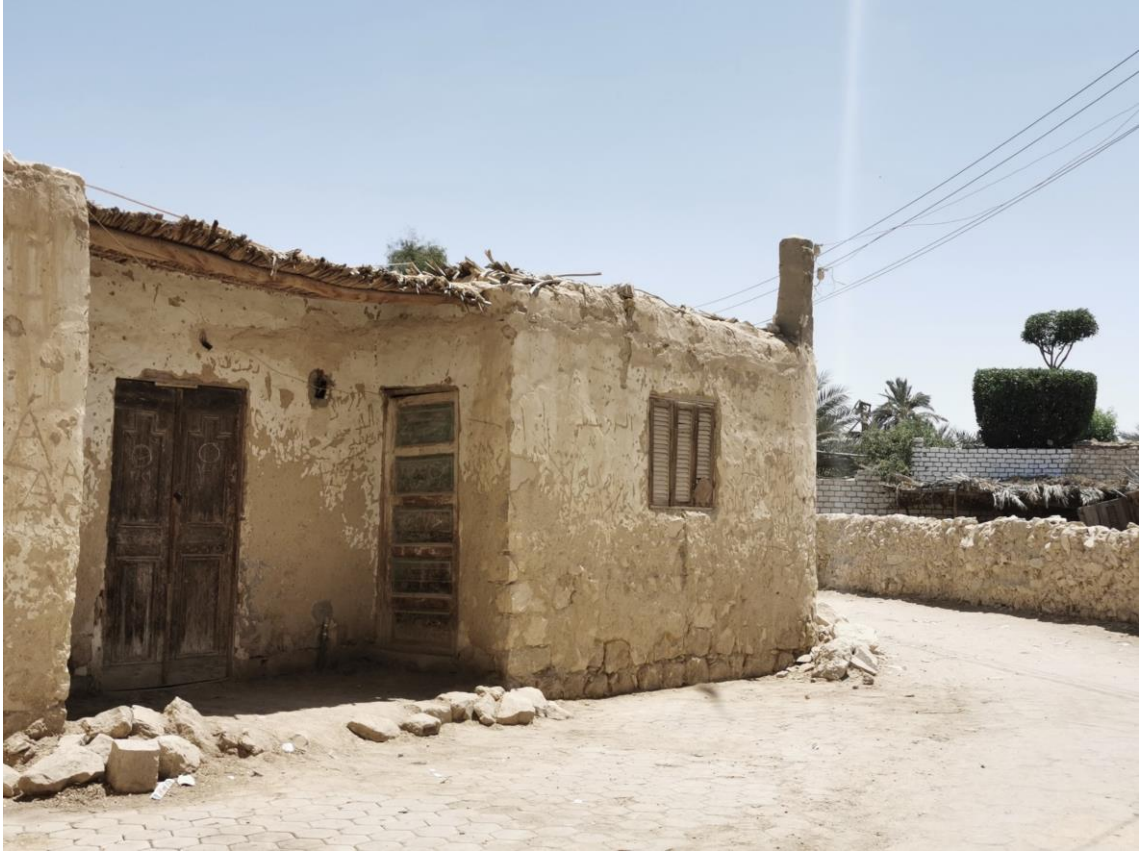
fig. 53. a traditional fallah house made of limestone and cement plastering
