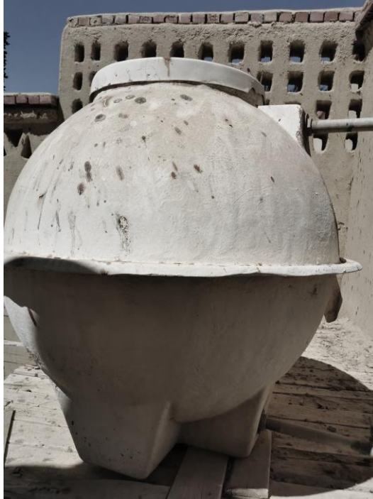
fig. 139. water silo on the rooftop
