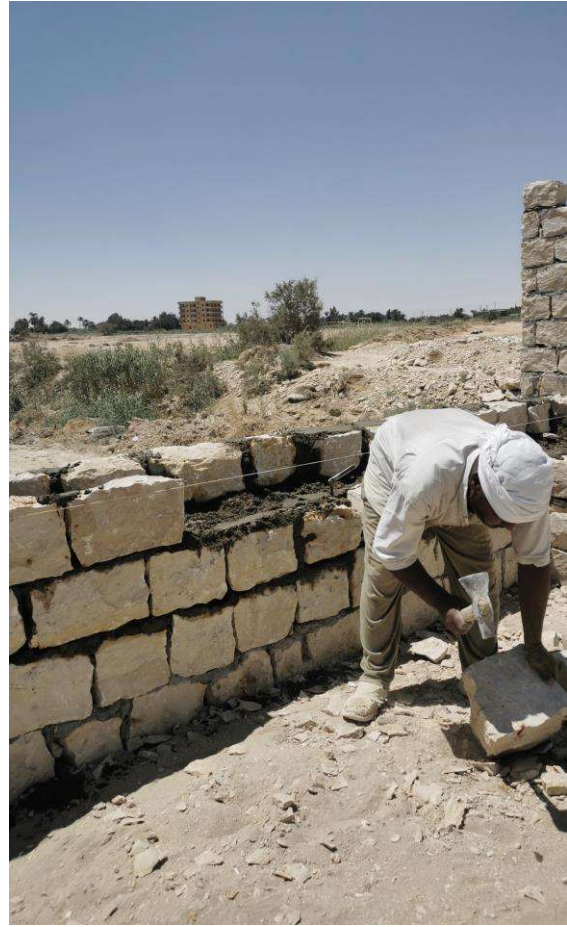
Fig. 70. hewing the „fayoumi stones“, Mansour's construction site
