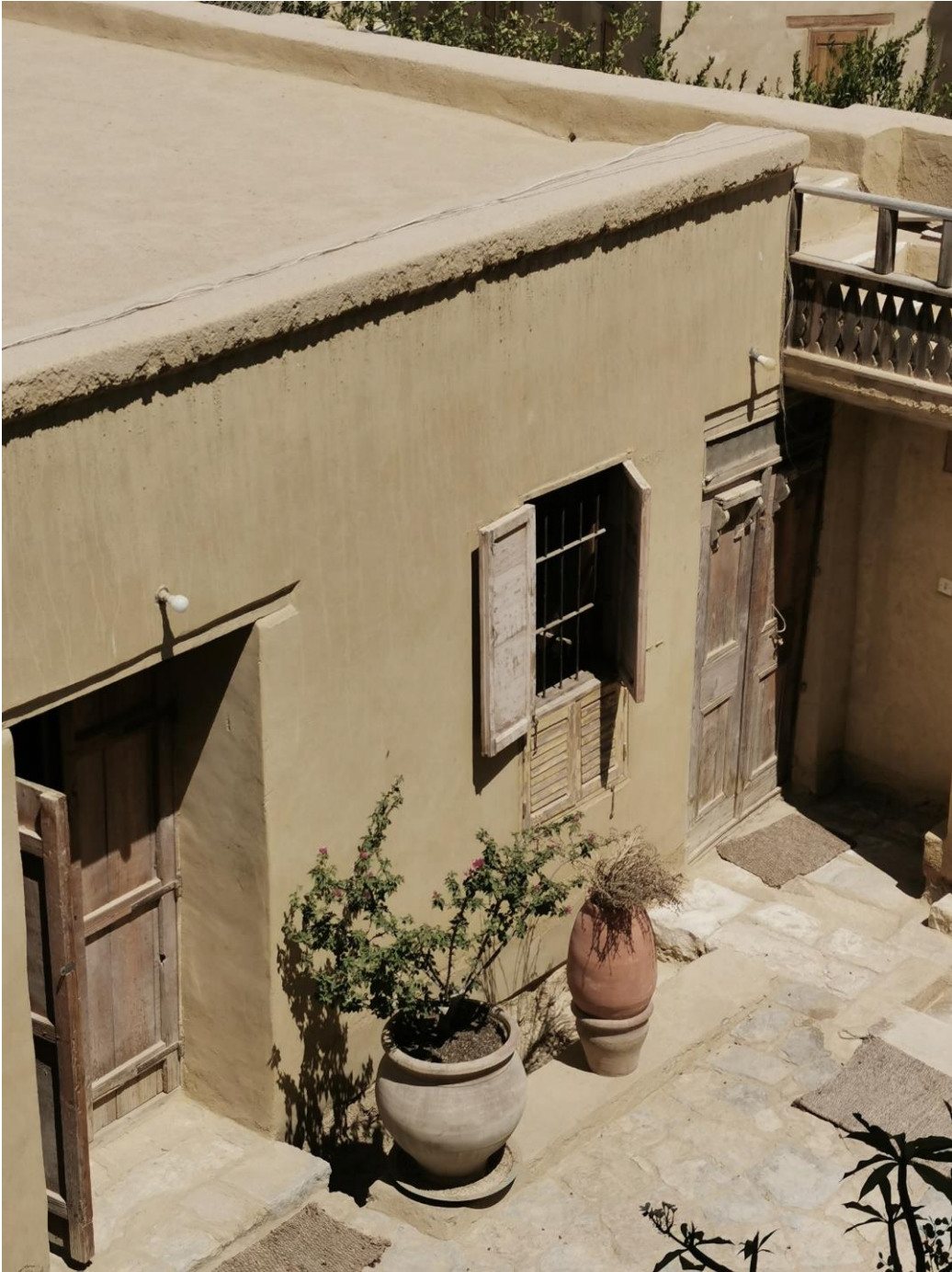
fig. 113. courtyard of the old part, Dr. Nabil's house
