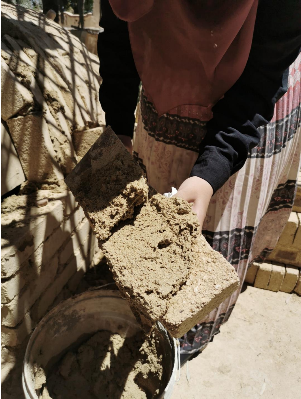
fig. 61. building with clay and mortar [ mouna ]
