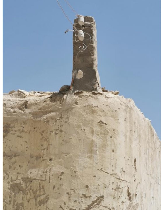
fig. 57. cement plastering of the fallah house
