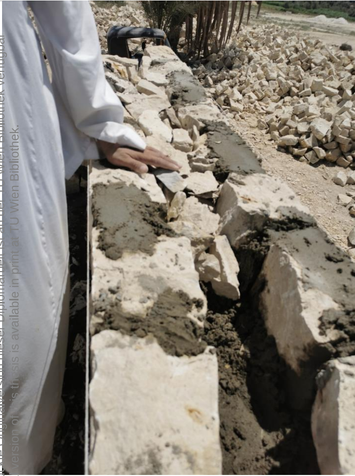
Fig. 69. shabaka, dabsch -construction, Mansour's construction site
