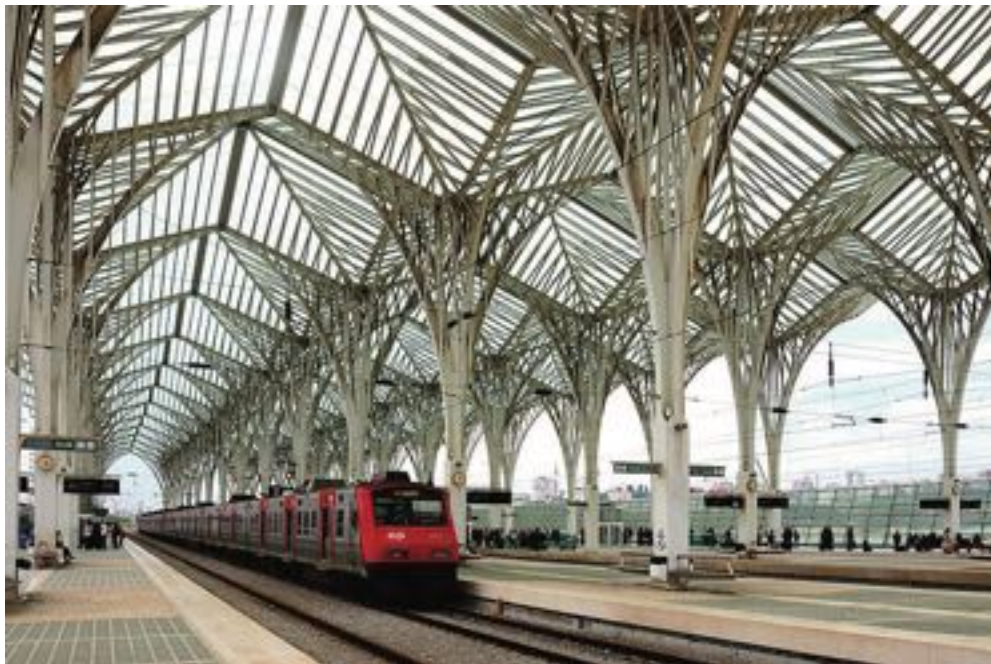
Station Oriente, Lissabon – Santiago Calatrava
