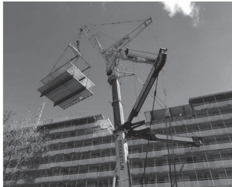
Figure 2: Deconstruction and new construction with reused materials within UIA Super Circular Estate project Kerkrade the Netherlands © E.Durmisevic 2021
