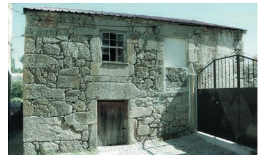
Abb.44: Steinbau in Santa Marinha
