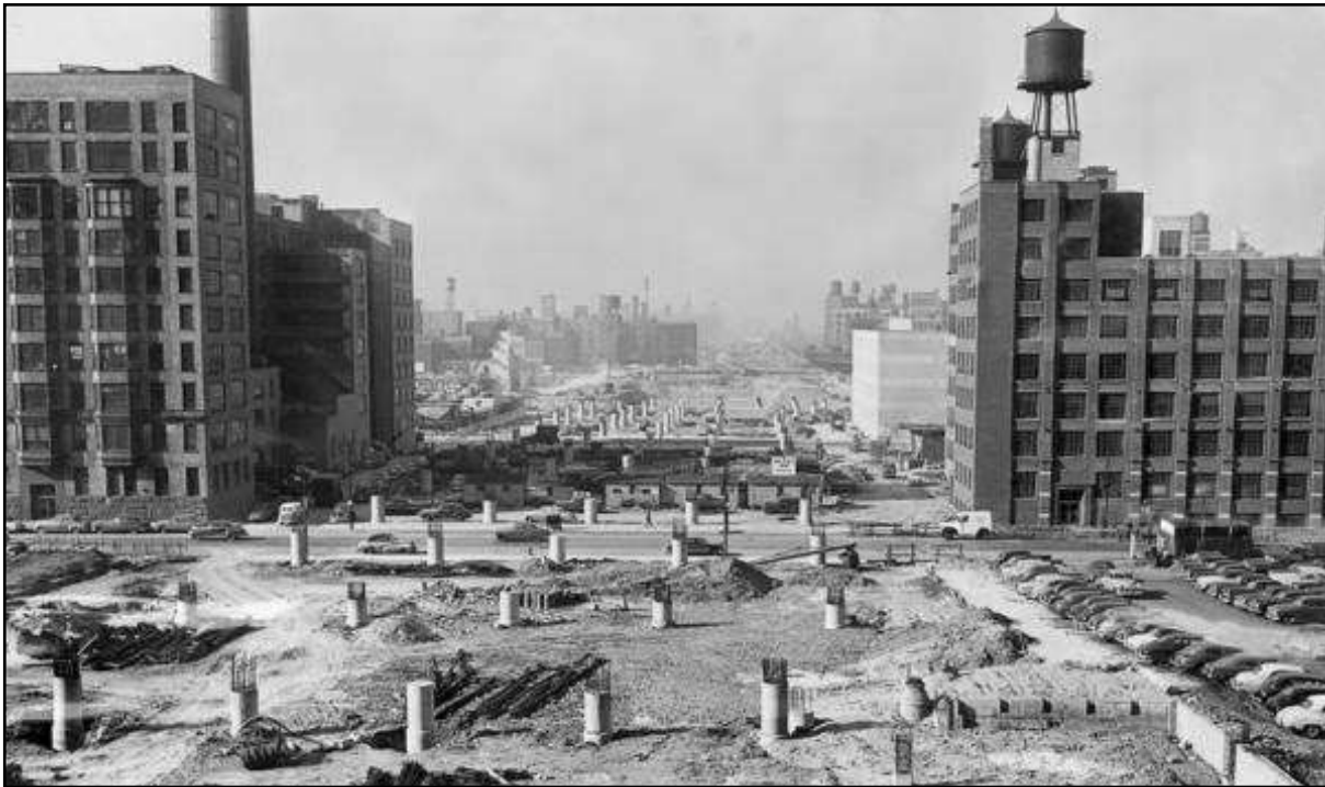
Abbildung 12: Bau des Congress Expressway, Quelle: Connecting the Windy City, 2013
